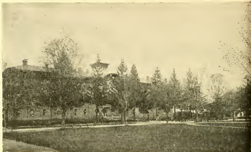
Rich Hall and Principal's Residence
