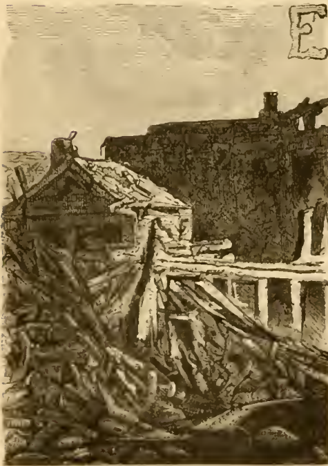
AFTER THE EARTHQUAKE.
