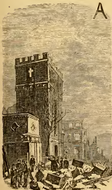
TRINITY CHURCH, BOSTON, DESTROYED.
