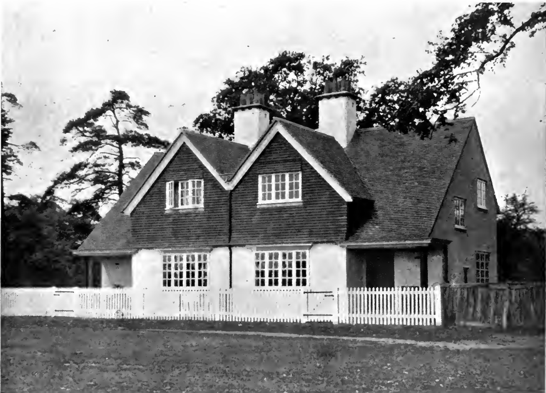
TWO COTTAGES AT RIPLEY, IN SURREY, COSTING £585 THE PAIR. MATERIALS: ROUGHCAST AND LOCAL TILE
