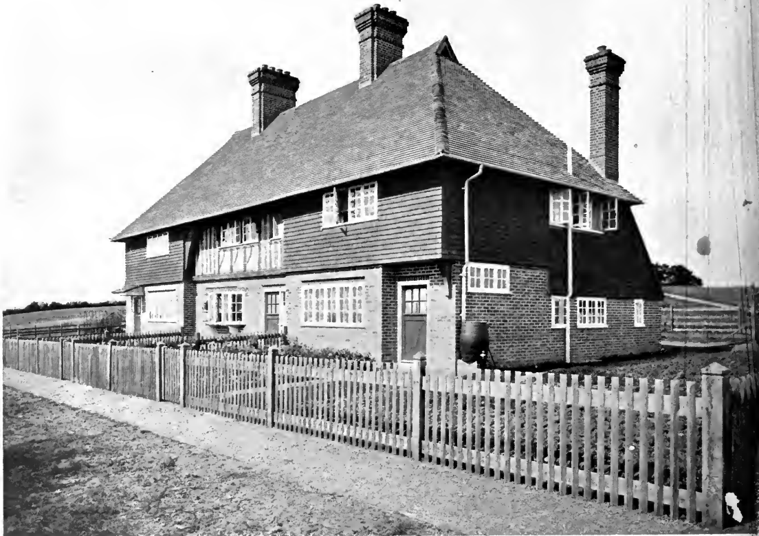
COTTAGES AT CHAPELWOOD MANOR. MATERIALS: RED BRICK, ODESSA OAK AND PLASTER, RED HANGING AND ROOF TILES
