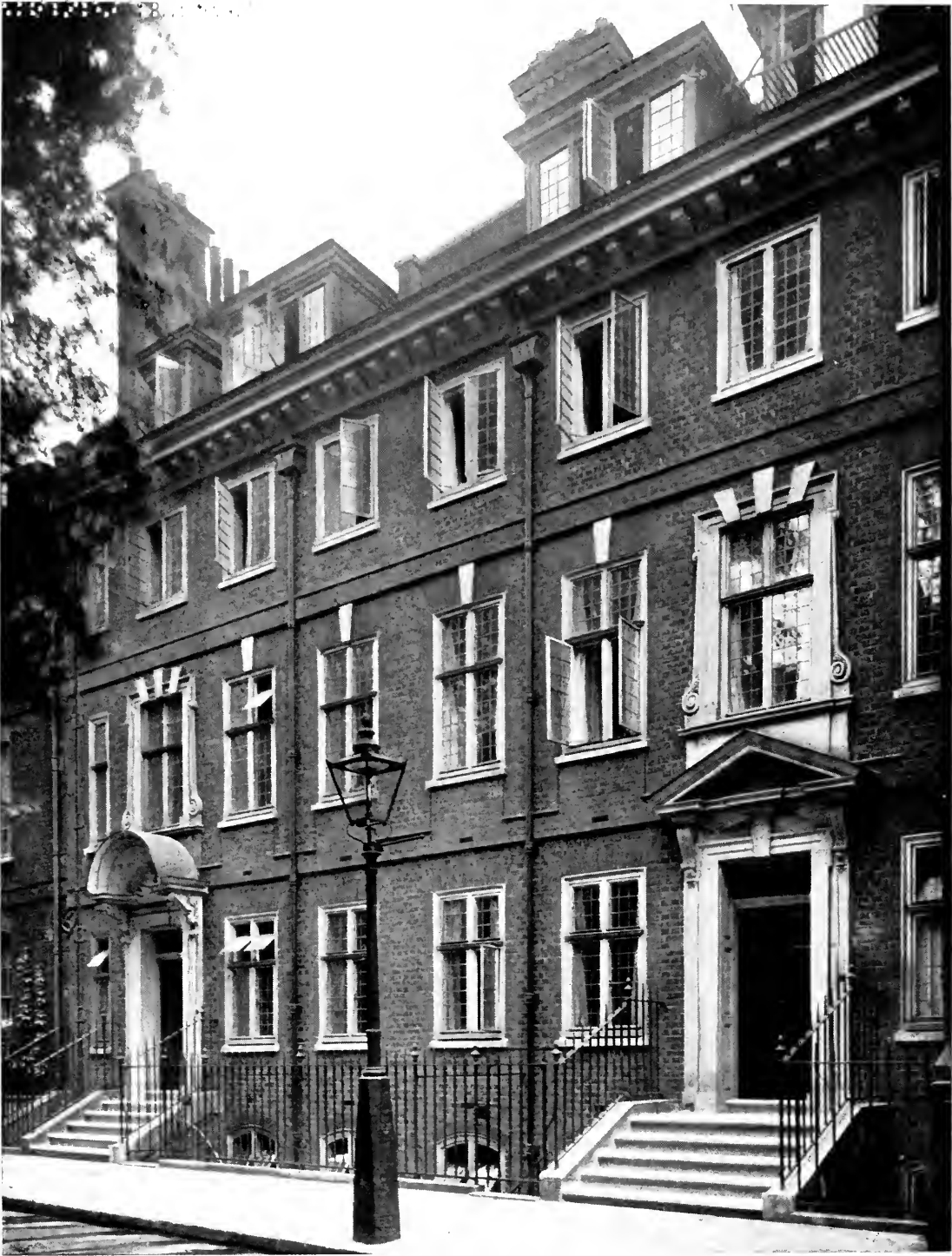
TWO URBAN HOUSES, 14 AND 15, GREAT COLLEGE STREET, WESTMINSTER, LONDON: BUILT ON THE SITE OF TWO OLD HOUSES WHICH WERE CONDEMNED. THEY ARE FACED EXTERNALLY WITH LIGHT RED DRESSINGS AND DARKER BRICKS FOR FILLING. THE ENTRANCE DOORS HAVE STONE DRESSINGS
