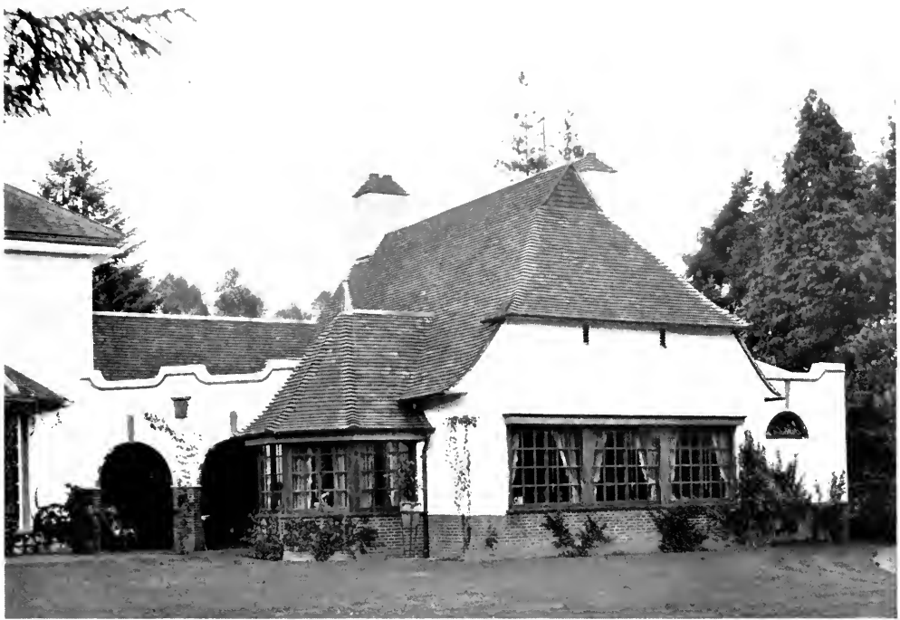
LINHOLME, HOLMBURY-ST.-MARY, DORKING. ADDITIONS FOR A. P. HOSKYN, ESQ. MATERIALS: THIN RED BRICK BASE, CEMENT ROUGHCAST WHITEWASHED, OLD HAND-MADE ROOFING TILES, THE WOODWORK OF ASH
