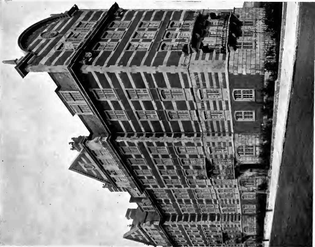
LANOVER HOUSE, ST. JOHN'S WOOD, LONDON. THESE FLATS ARE BUILT OF RED BRICK AND PORTLAND STONE, WITH A ROOF OF GREY-GREEN SLATES. THE DRAWING WAS CARRIED OUT BY T. E. JAGO. THE PLAN REPRESENTS TWO SUITES OF ROOMS, WITH THE CORRIDOR OF EACH FLAT, LIGHTED FROM AN AREA. THE KITCHENS ARE WELL PLACED IN THEIR RELATION TO THE BEDROOMS AND OFFICES OF THE SERVANTS' QUARTERS. THE RENTS, INCLUDING RATES AND TAXES, RANGE FROM £188 TO £240 PER ANNUM
