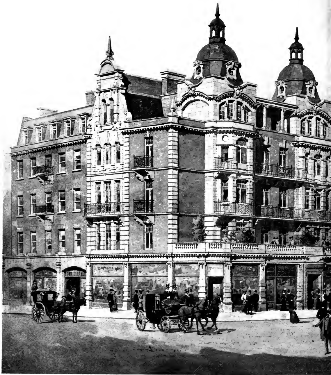
BLOCK OF FLATS, ST. GEORGE'S TERRACE, GLOUCESTER ROAD, LONDON, SHOWING THE ELEVATION WITH Paul Hoffman
