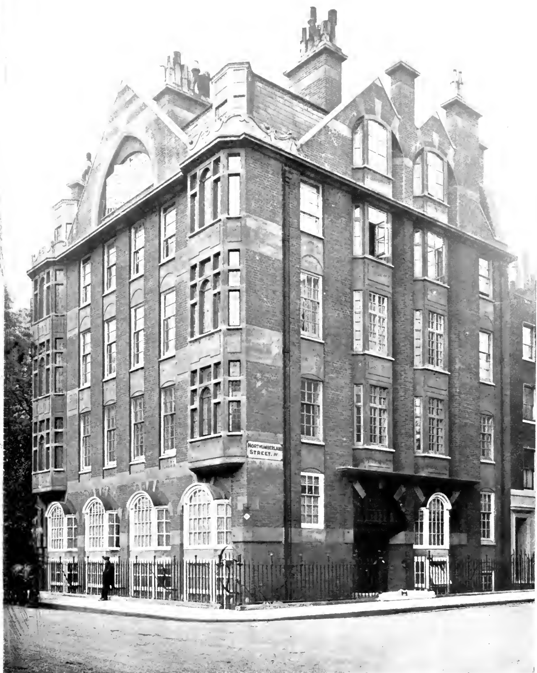
LUXBOROUGH HOUSE, NORTHUMBERLAND STREET AND PADDINGTON STREET, LONDON, W. THIS BLOCK OF FLATS SHOWS THAT EXCELLENT DESIGN AND SOUND WORKMANSHIP CAN BE COMBINED WITH THE STRICTEST ECONOMY IN MATTERS OF EXPENSE
