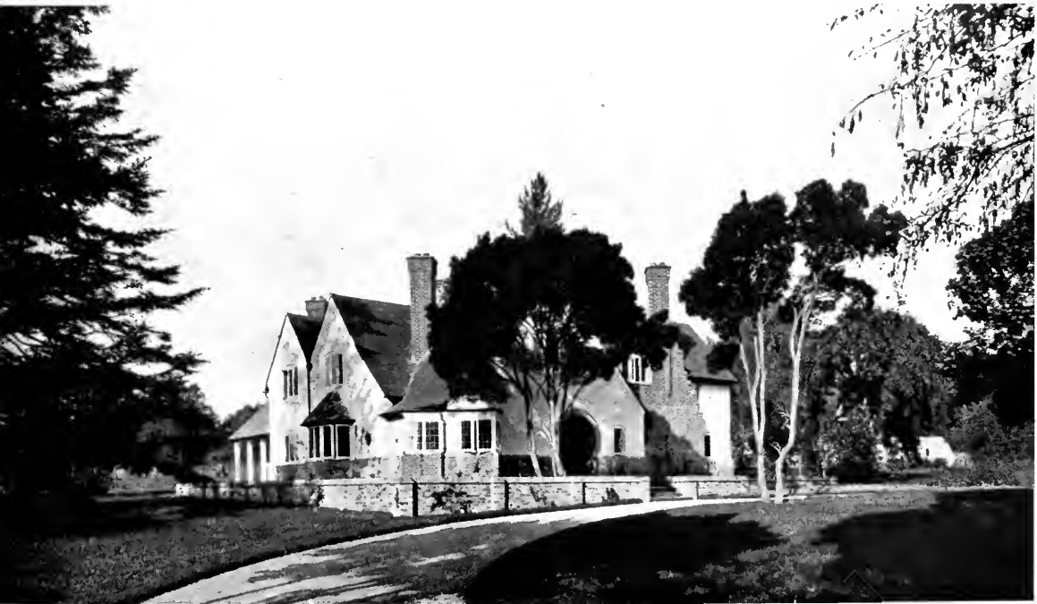
DOVER, POLING, NEAR ARUNDEL, SUSSEX. THE LOWER PARTS OF THE WALLS ARE FACED WITH RED BRICKS OF VARIED COLOUR, WHILE THE UPPER PART IS COVERED WITH CEMENT ROUGHCAST
