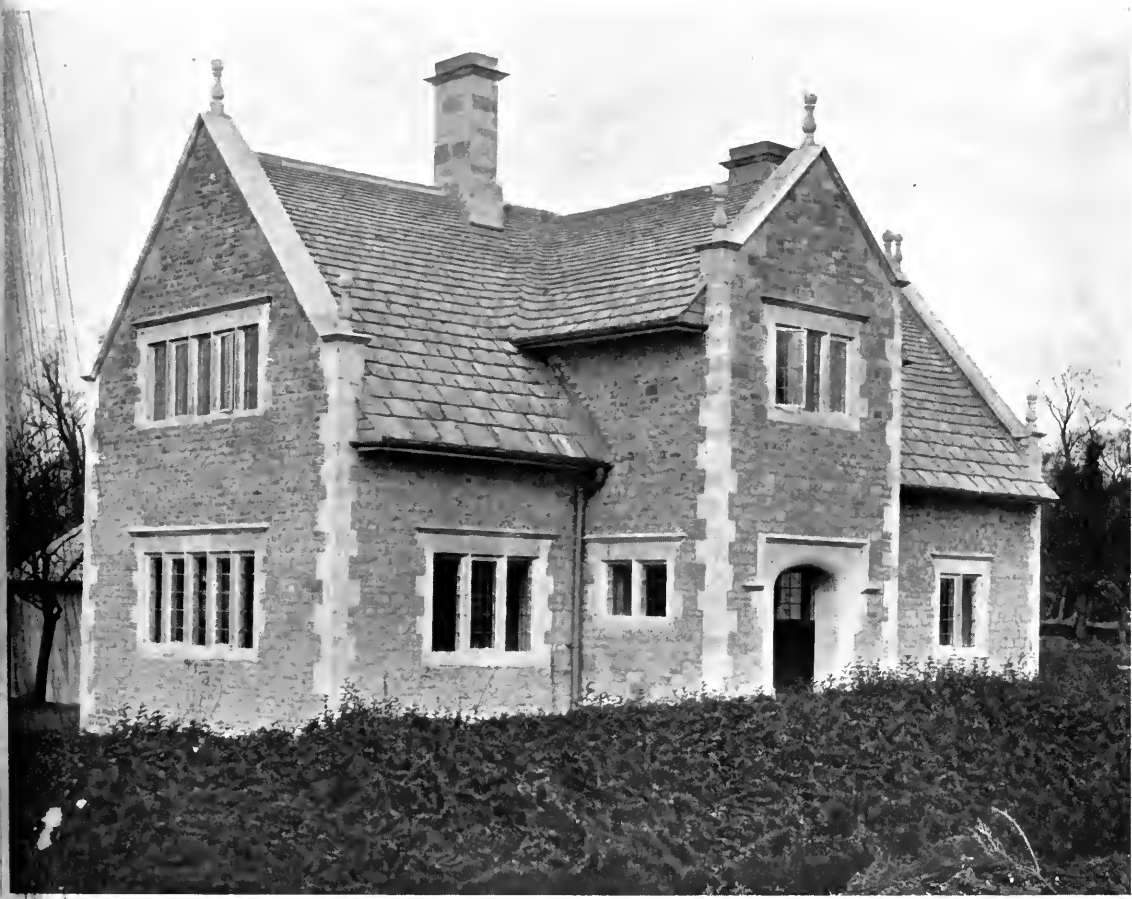
COTTAGE AT APETHORPE, BUILT FOR L. BRASSEY, ESQ. MATERIALS: EDITH-WESTON STONE AND COLLY-WESTON SLATES
