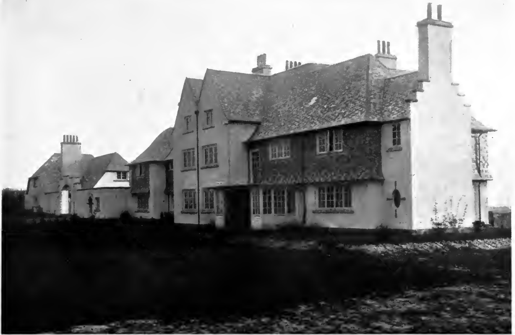
HOUSE AT NORTH BERWICK, VIEW FROM THE S.W. BUILT OF LOCAL WHINSTONE HARLED AND WHITEWASHED, WITH SLATE-HANGING AND ROOFS OF SCOTCH SLATES
