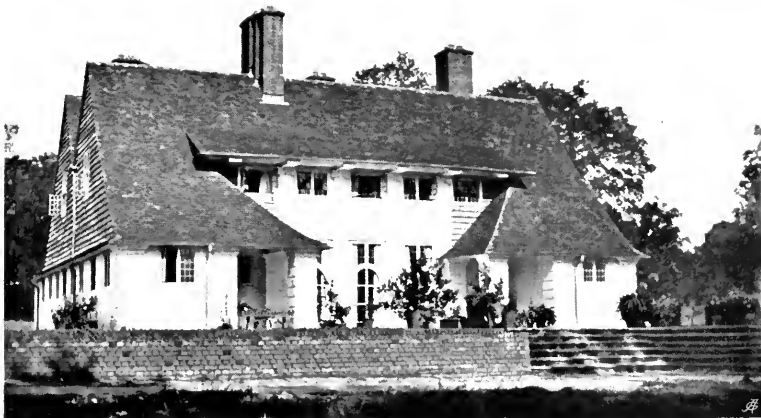
HOMWOOD, KNEBWORTH, HERTFORDSHIRE, THE SEAT OF THE DOWAGER COUNTESS OF LYTTON. MATERIALS: TILES FOR THE ROOF AND BRICK AND WOOD FOR THE WALLS. SOUTH-EAST SIDE
