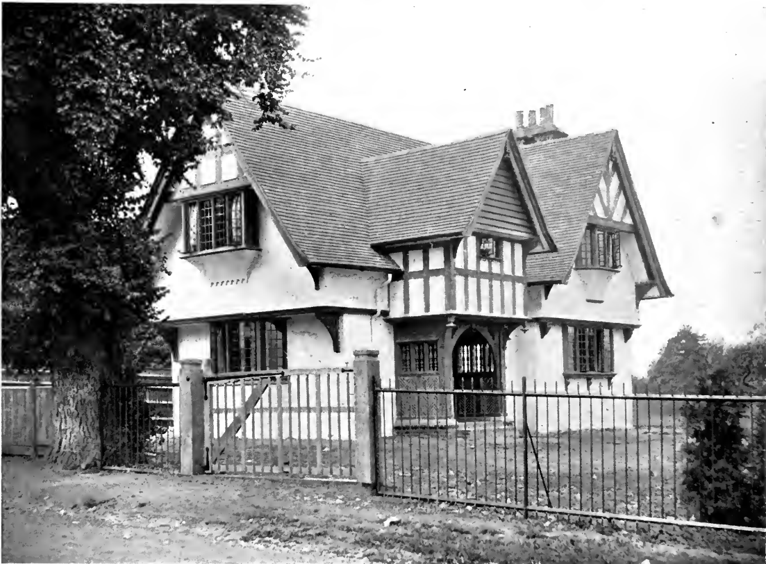
COTTAGE AT CHISLEHURST. THE WINDOWS AND THE EXTERNAL WOODWORK ARE OF OAK, THE WALLS ARE WHITEWASHED, THE BUILDING IS ROOFED WITH KENT TILES
