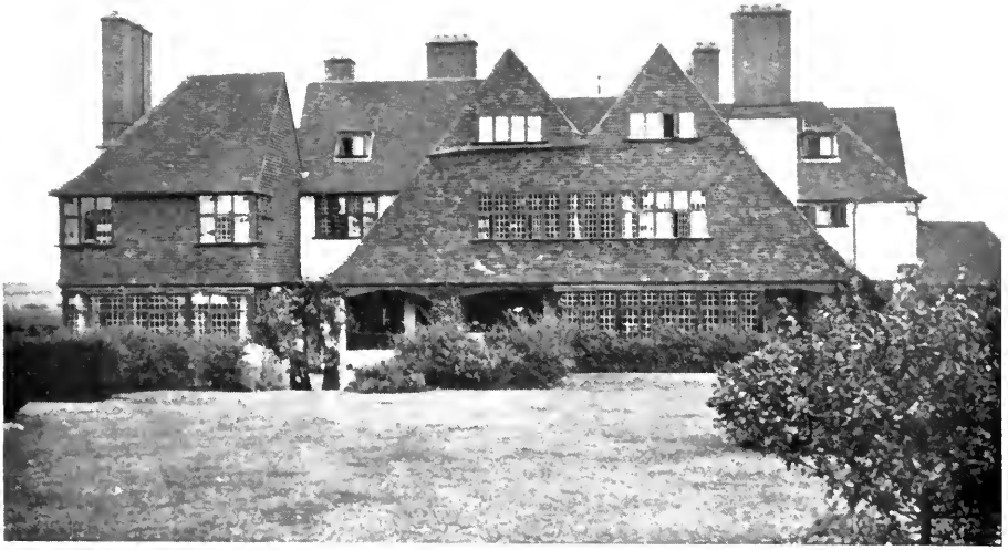
BERRYDOWN, HAMPSHIRE. MATERIALS: BRICK AND TILE HANGING, OAK WINDOWS AND LEADED LIGHTS
