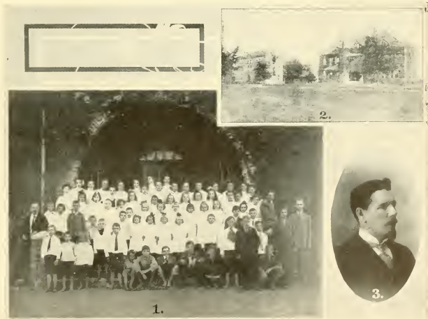
1. The Children 2. The Buildings 3. The Superintendent, George Dunglinson
