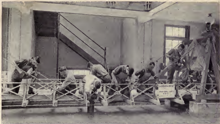
Military engineering will become a popular and necessary part of the curricula of our colleges and technical institutes. A class in suspension-bridge work at Wentworth Institute, Boston, Massachusetts
