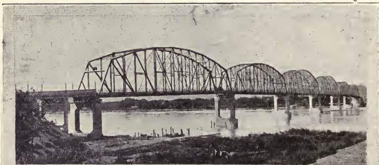
BRIDGE OVER MISSOURI RIVER AT PIERRE-FORT PIERRE.
