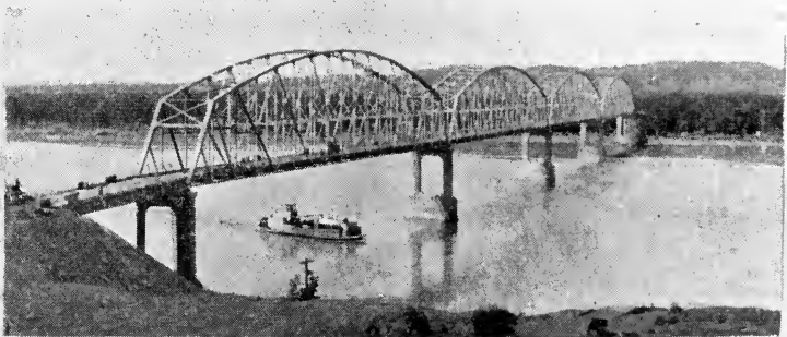
BRIDGE OVER MISSOURI RIVER AT CHAMBERLAIN
