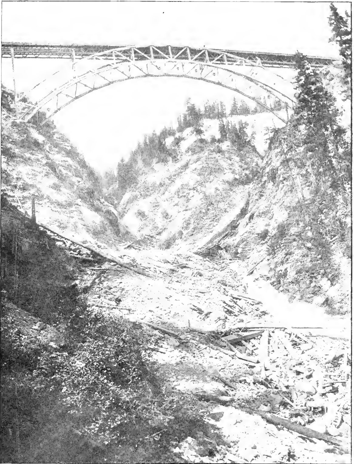
ONE OF THE MANY RAILROAD BRIDGES IN THE CANADIAN ROCKIES.
