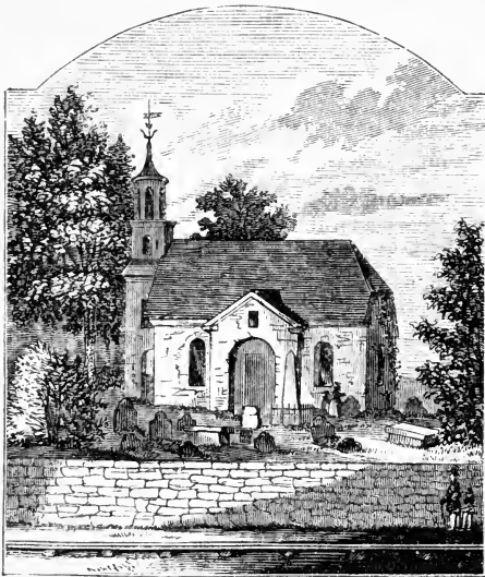
SOUTH-EAST VIEW OF SWEDES' CHURCH AT WILMINGTON.
