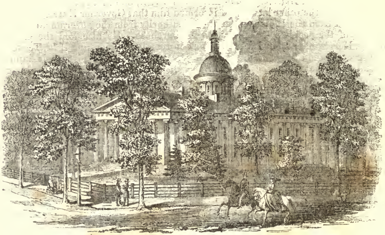
View of the State House, from Washington-street, Indianapolis.
