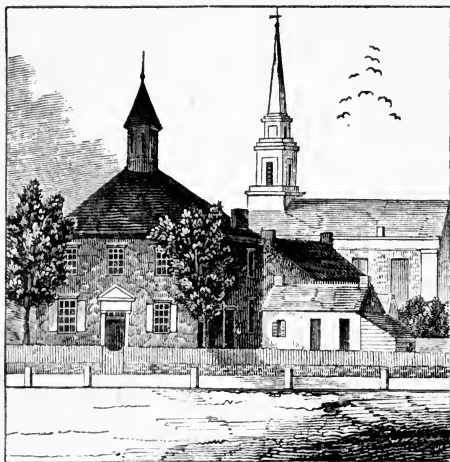
OLD STATE HOUSE, CHILLICOTHE.
