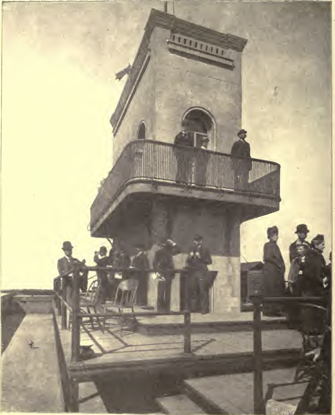
ON THE AUDITORIUM TOWER—HOME OF THE WEATHER BUREAU IN CHICAGO. Here, 320 feet above the ground, the observations are made which help to forecast the weather for the Great Lakes region. The small tower with the encircling balcony is the signal service office, and the instruments are on the roof.
