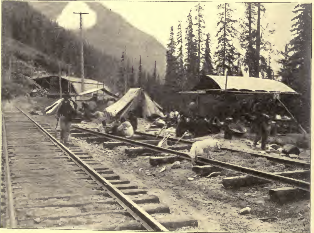
RAILWAY CONSTRUCTION IN THE MOUNTAINS.
