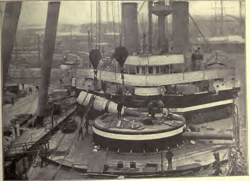
PLACING A BIG GUN ON BOARD A BATTLESHIP.
