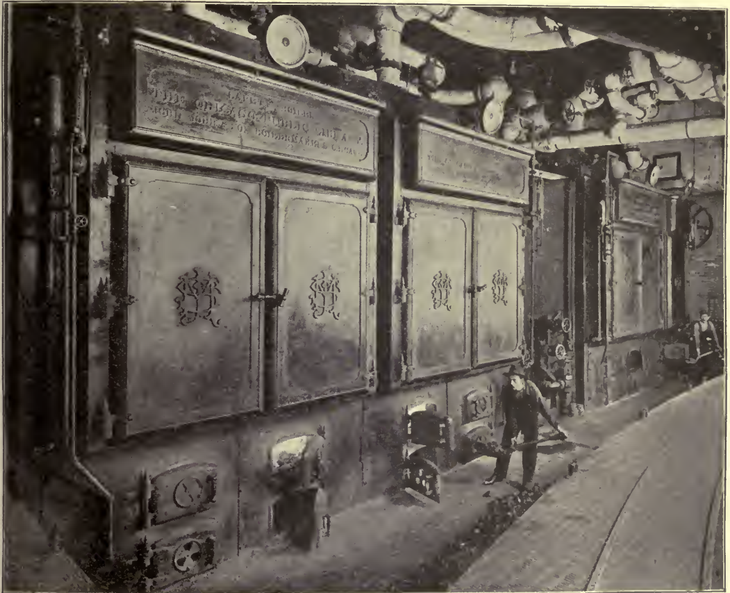
FIRING BY HAND—FURNACE ROOM OF THE CHICAGO PUBLIC LIBRARY.
