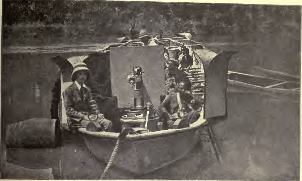
ARMORED BOAT FOR RIVER SERVICE IN CENTRAL AFRICA.
