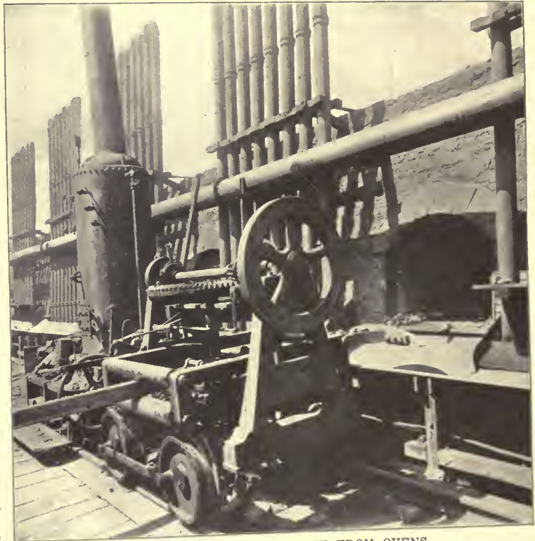
DEVICE FOR REMOVING COKE FROM OVENS.
