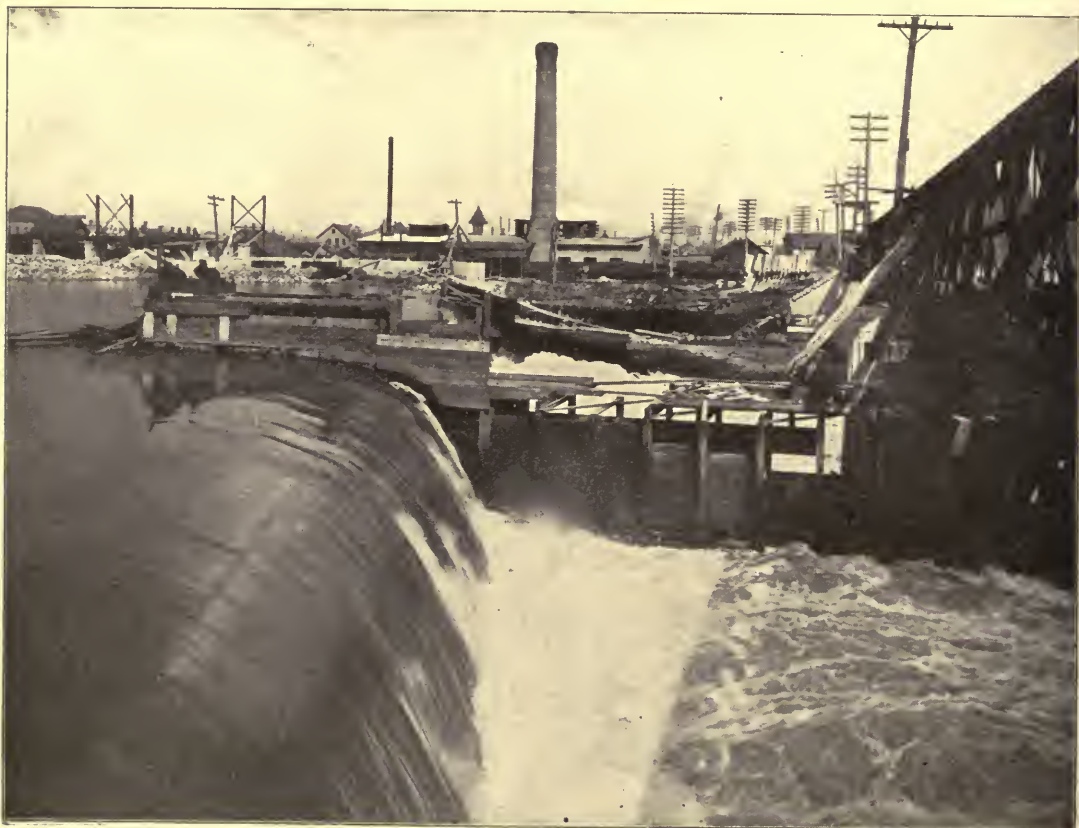
DAM AT LOCKPORT, ON THE CHICAGO DRAINAGE CANAL.
