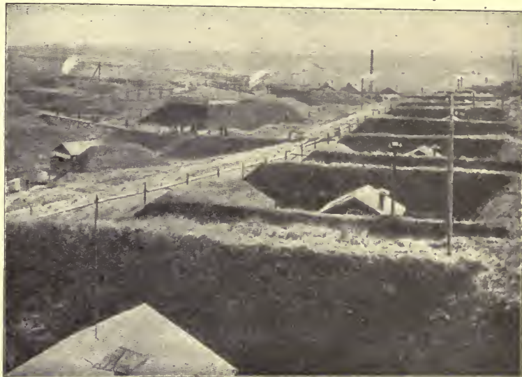
FACTORY FOR HIGH EXPLOSIVES, SHOWING EARTHEN WALLS, TO PROTECT AGAINST DISASTERS.
