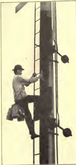
Carrying night lanterns to the top of a railway signal post.
