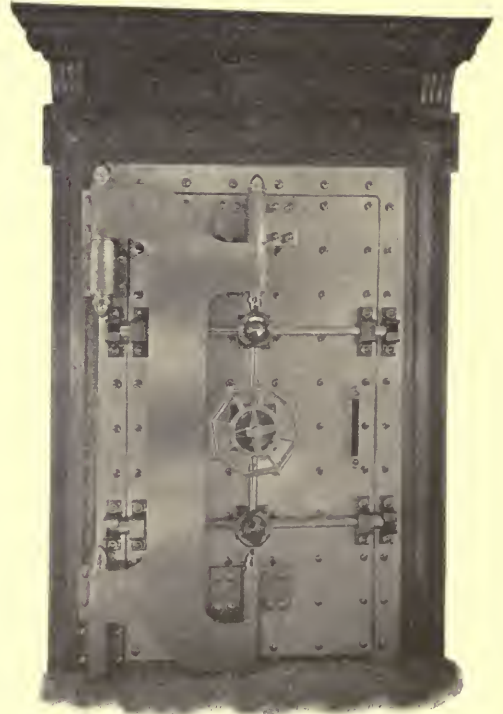
BANK VAULT DOOR CLOSED.
