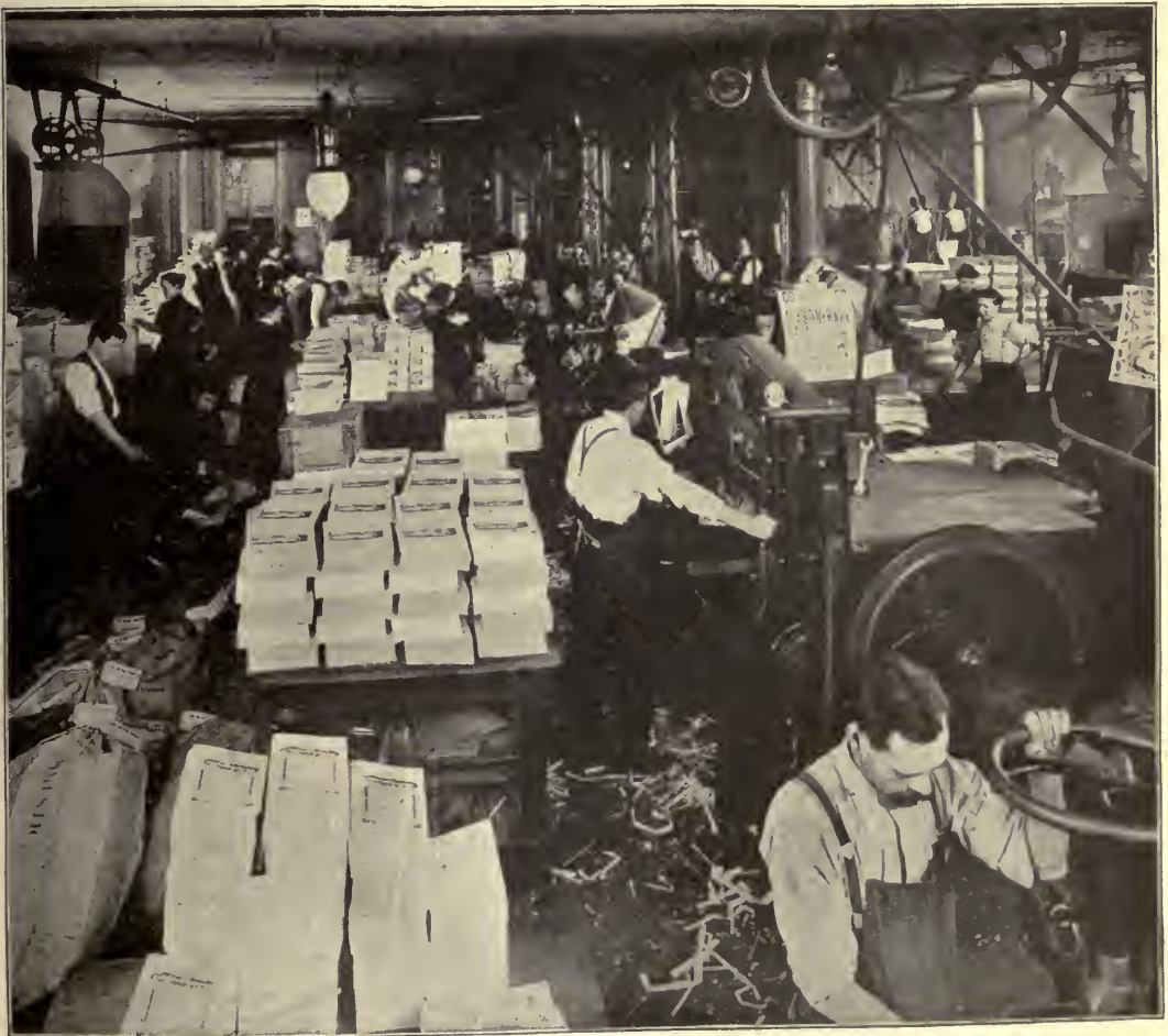
TRIMMING AND MAILING MAGAZINES IN A BINDERY.
