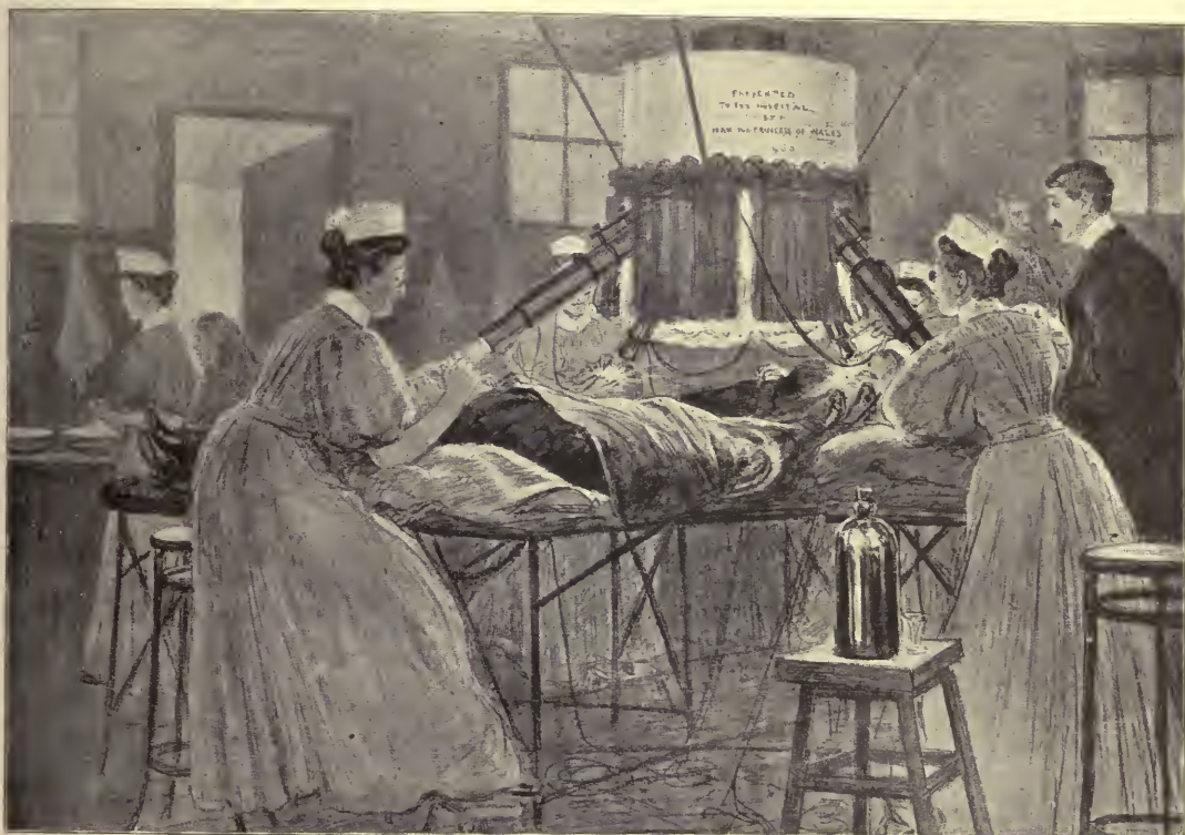
APPLICATION OF THE LIGHT CURE IN A LONDON HOSPITAL.
