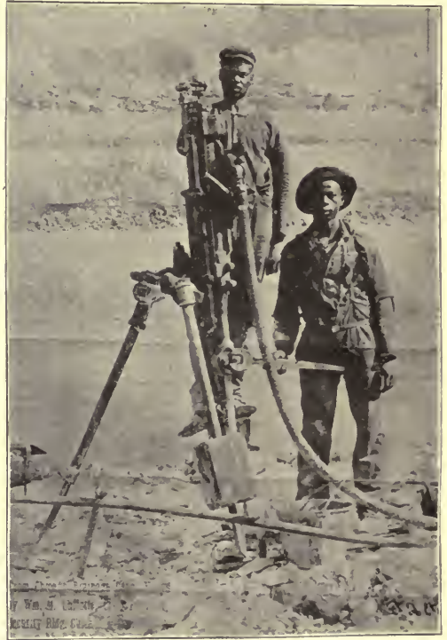
COMPRESSED-AIR DRILL, CHICAGO DRAINAGE CANAL.
