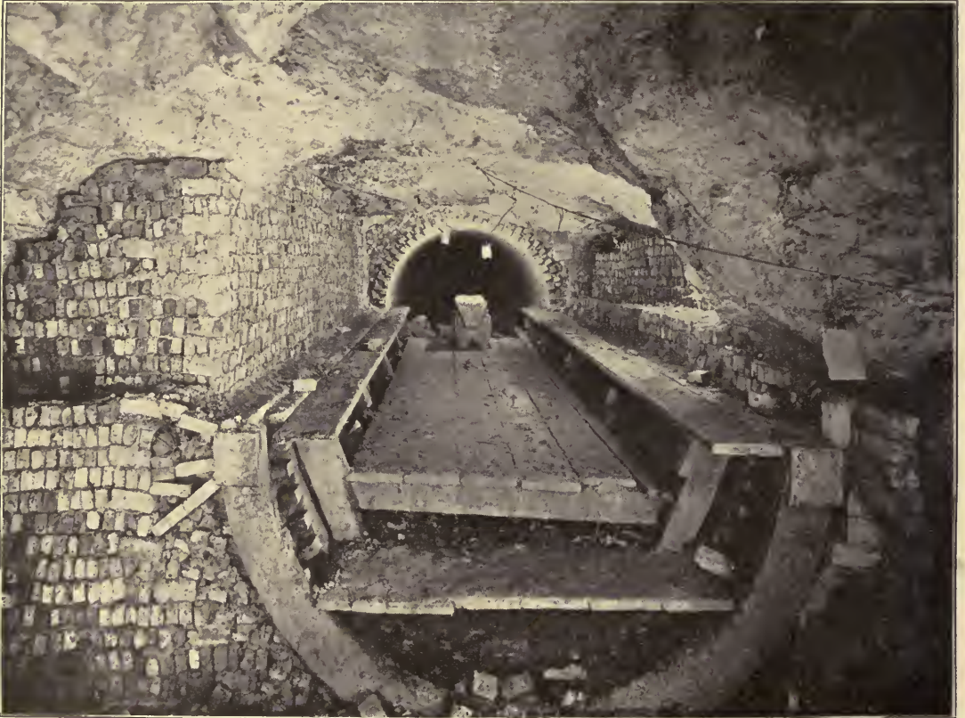
BUILDING A POWER-TRANSMISSION TUNNEL FROM A GREAT CANAL.
