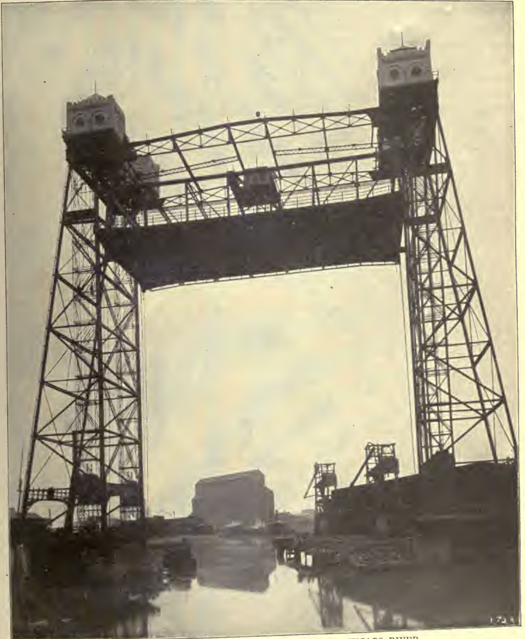
HALSTED STREET LIFT BRIDGE OVER THE CHICAGO RIVER.
