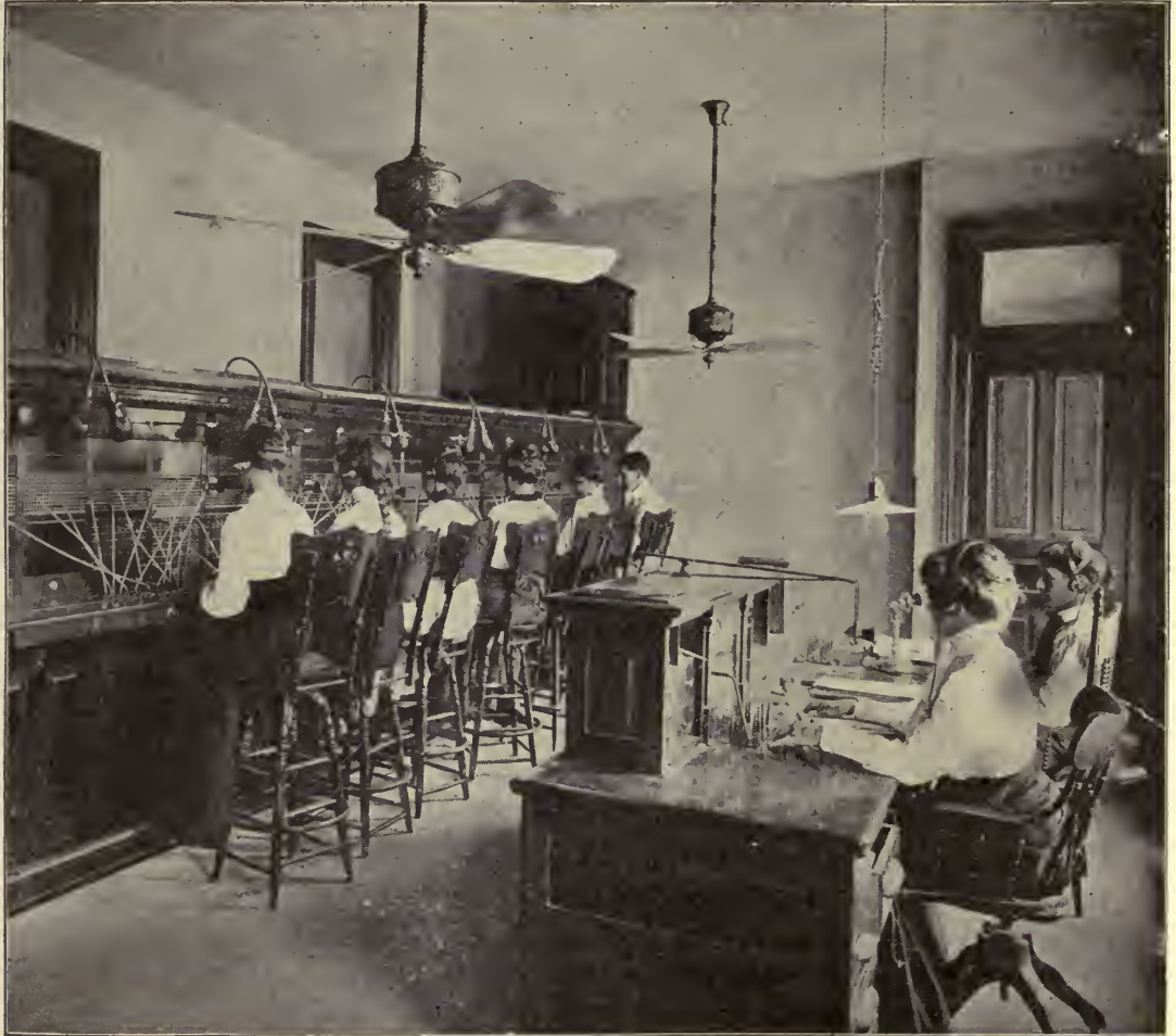
PART OF OPERATING ROOM IN A TELEPHONE EXCHANGE.
