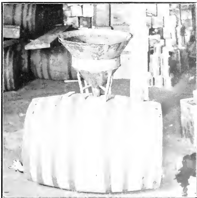
Fig. 24. The Dadant strainer for barrels.
