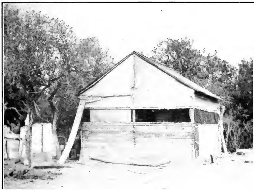
Fig. 55. Honey-house built with ample ventilation for extracting.
