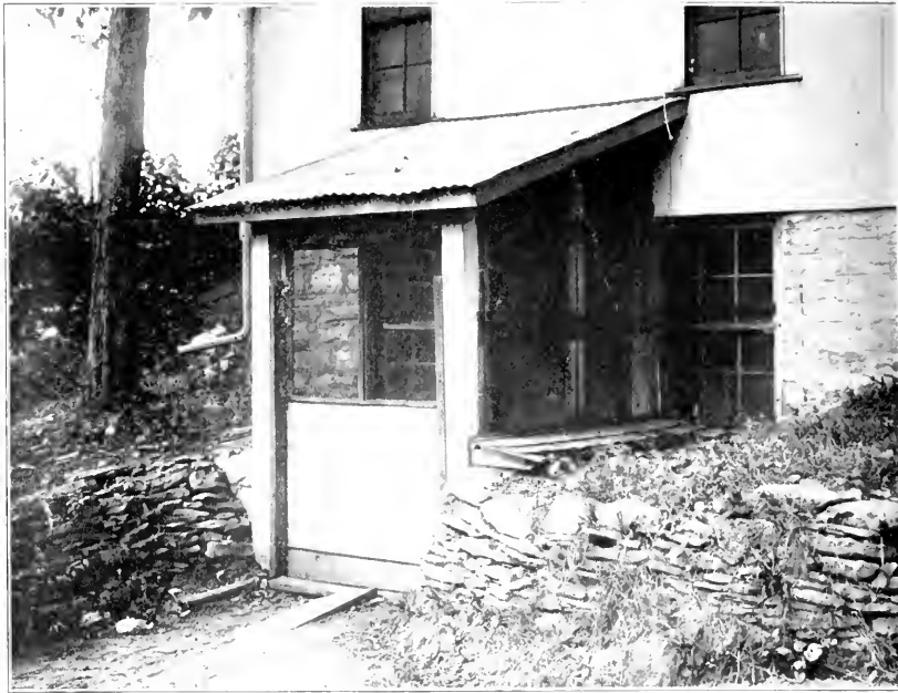
Fig. 51. Screened entry to the honey-house that will keep the bees out.
