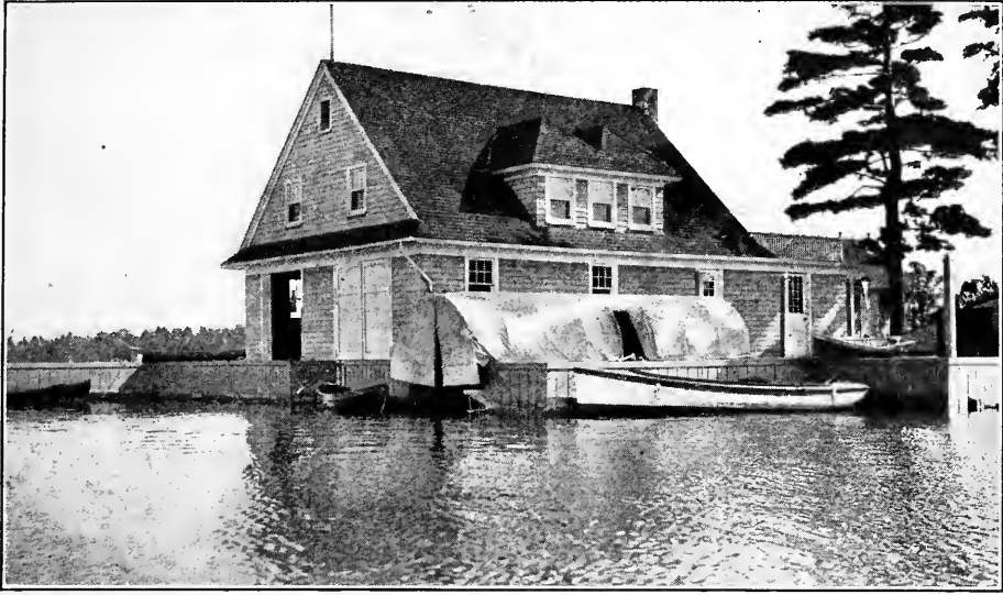
A SLOPING CANVAS ROOF WILL KEEP OUT THE DAMPNESS AS EFFECTUALLY AS WILL ONE MADE OF TIMBERS AND SHINGLES OR TILE
