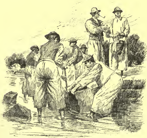
"REPAIRING THE BROKEN LEVEES." (p. 254.)
