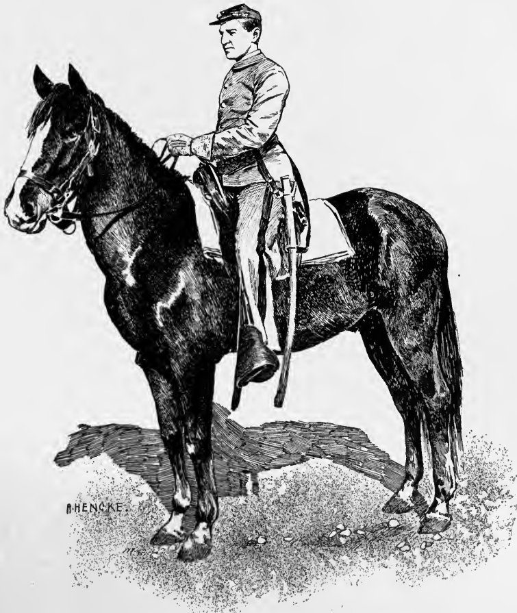
READY FOR DRILL.
