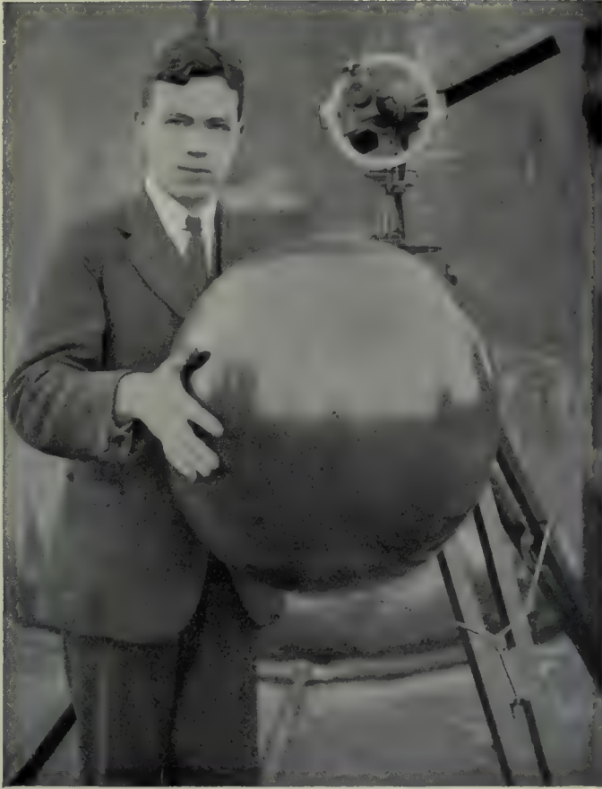
A PILOT BALLOON READY TO BE RELEASED
