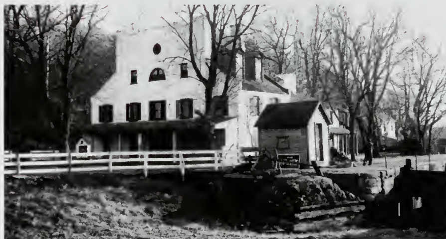
Photograph 44: The north front of the Tavern, completed in 1832, and built of brick, like the addition at the south end, completed at the same time. The porch is a comparatively recent addition and is to be removed. In the right foreground are the Lock (No. 20), gate closed, butterfly valve open, one of the slots for temporary dam, the cribbing between the lock and the opening for the spillway, and the much newer shack for the lock tender.
