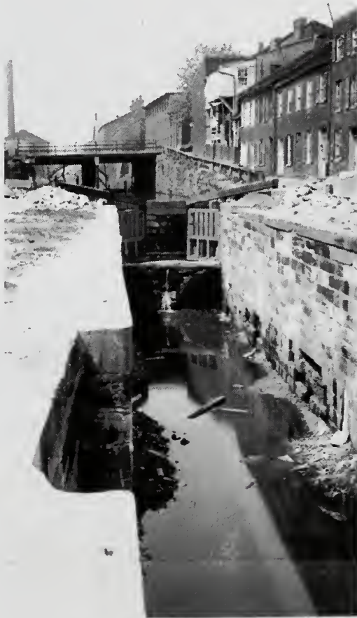
Photograph 1: Swing Gates. Lock No. 4, in Georgetown, shows also the character of the Lock masonry and the dam at head of the Lock. Composed of heavy planks lowered into slots cut in the stone. This served to hold back water during repairs. The curve of the arch of the Wisconsin Avenue Bridge appears in the background.
