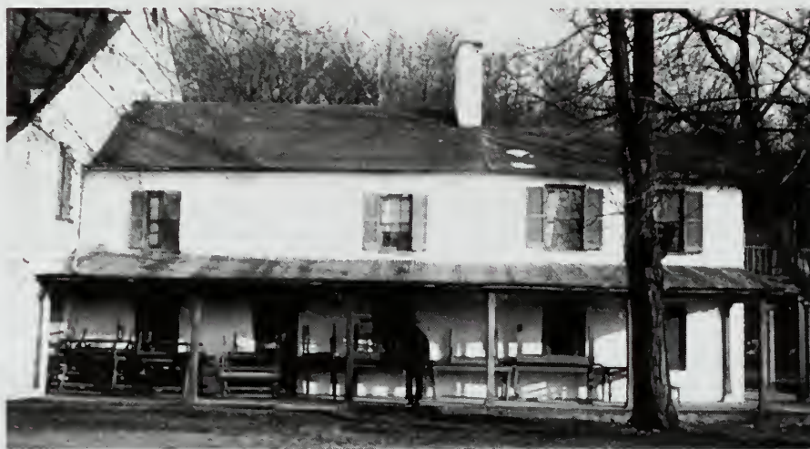
Photograph 43: The Great Falls Tavern. The central portion, from the chimney to the higher wall, was begun in 1828 as a lock tender's house, and is of the typical stone construction.
