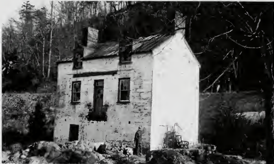
Photograph 39: House at Lock No. 16. The first house built from the second or 1836 specifications. It stands on a rock ledge well above the lock. This building cannot be used without considerable reconstruction of the interior.
