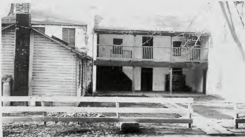
Photograph 46: The north side of the Tavern. On the left is the wooden kitchen added in 1926 to replace a similar structure. In the verandah or gallery, appears the slope of the outside stair that was the only means of communication between the ground and first floors. The central part is the 1828 building.
