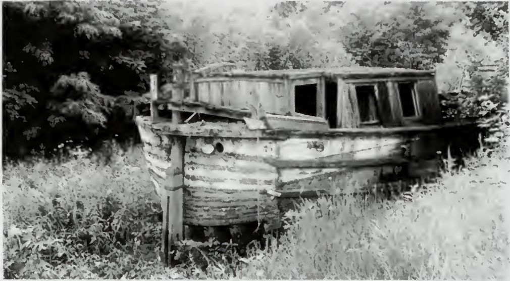
Photograph 59: Stern, cabin, rudder post, quarter-deck and one post of taffrail. Also curved planking on upright timbers. Construction of bow is similar.
