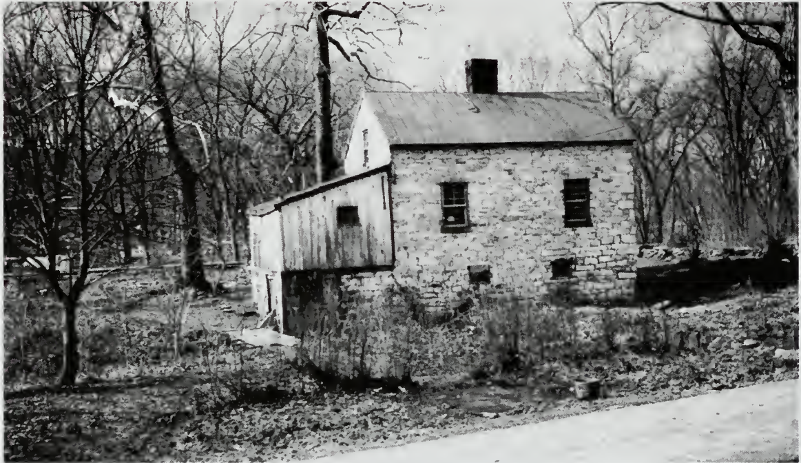
Photograph 28: House at Lock No. 6 has kitchen built partly on projecting stone walls. The line of the lock appears in the background. This photograph shows excellently the texture of the old masonry as well as the adaptation of the specified type to differing conditions of site.
