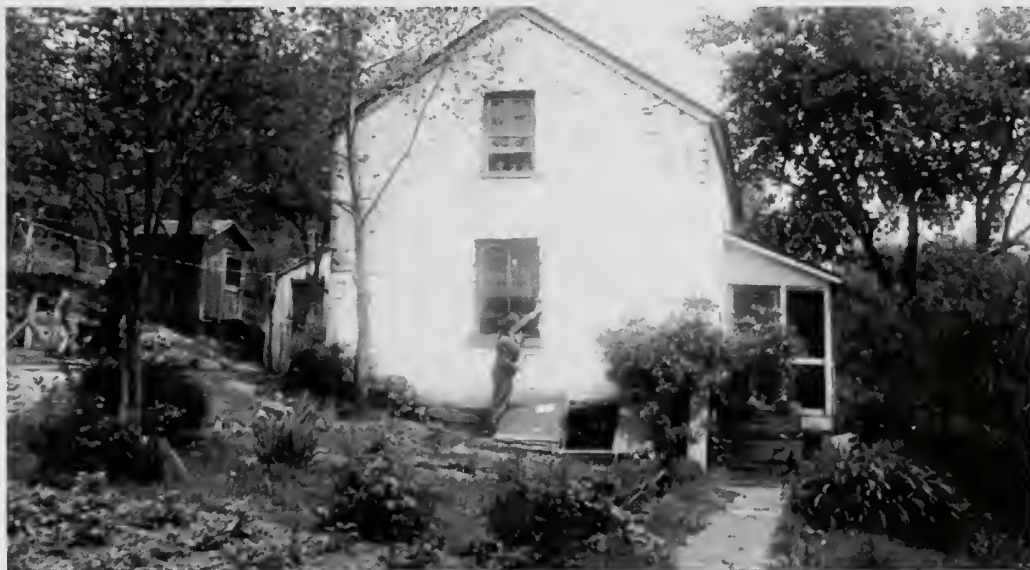
Photograph 34: The same house, showing bulkhead entrance to cellar, typical whitewashed masonry and the corner of the wooden kitchen addition. This building is being restored in the same manner as the houses at Locks No. 7 and No. 5.
