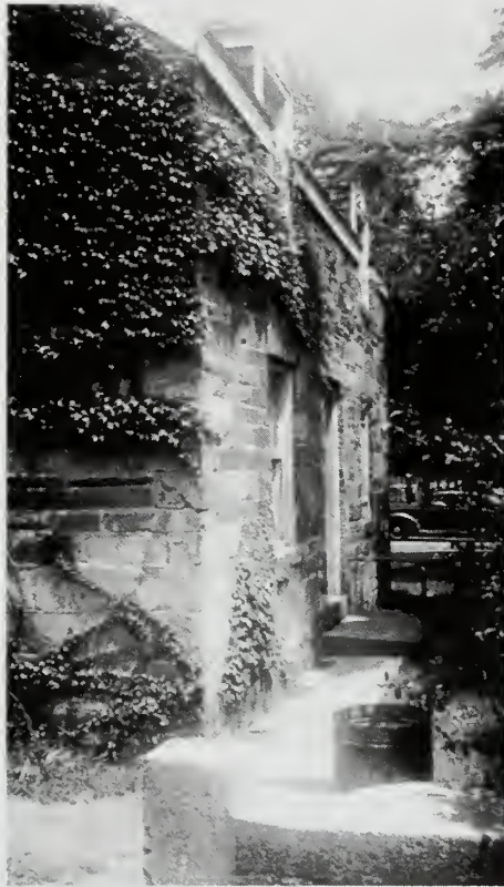
Photograph 22: Lock House from canal once connecting Potomac River through Tiber Creek (see map) with the Eastern Branch (Anacostia) and converted in 1878 into a sewer. The house was moved about twenty years ago to this site at 17 th Street and Constitution Avenue. It is like the C & O Lock houses in design and construction. Work on this older canal began in 1792.
