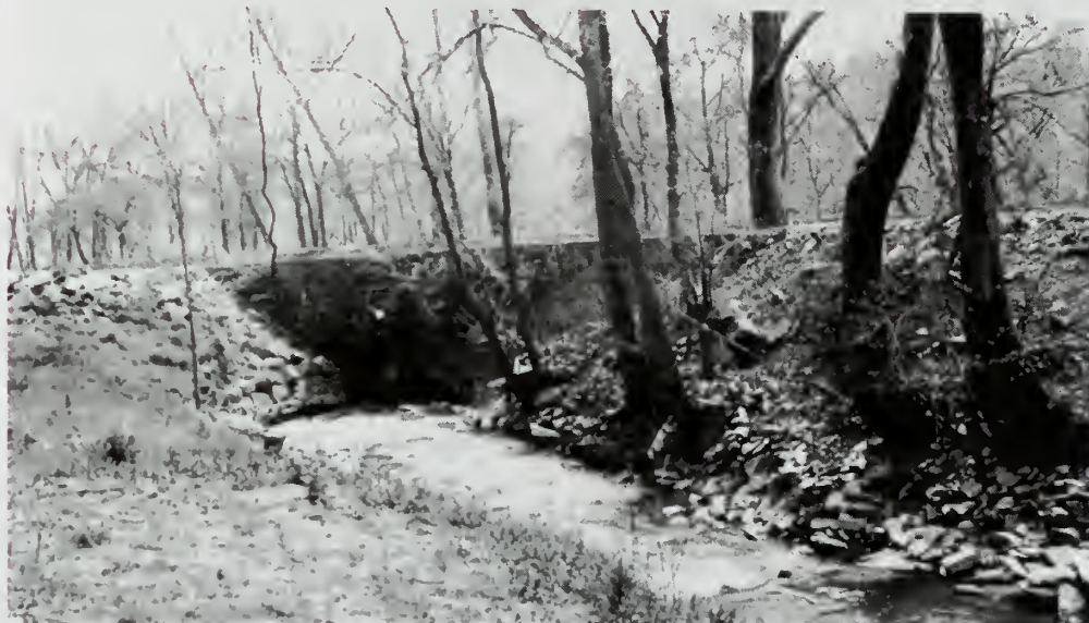
Photograph 12: Culvert below Lock No. 5.
