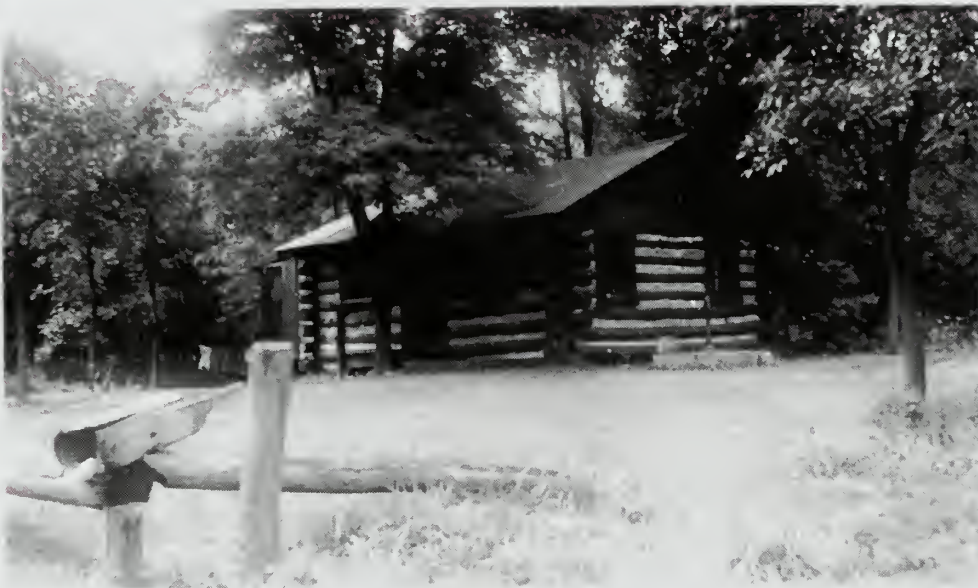
Photograph 52: New log house on foundations of Lock Tender's house at No. 23, burned a few years ago. Although the building is out of character with the other Canal structures it will continue in use.
