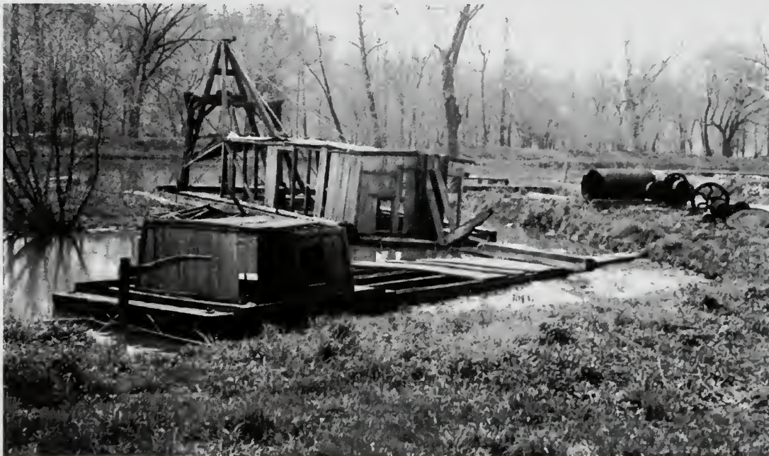
Photograph 64: The Canal “Graveyard”: An abandoned work barge and the dismantled dredge with boiler and some of the machinery lying on the shore. This is between Chain Bridge and Lock No. 5.
