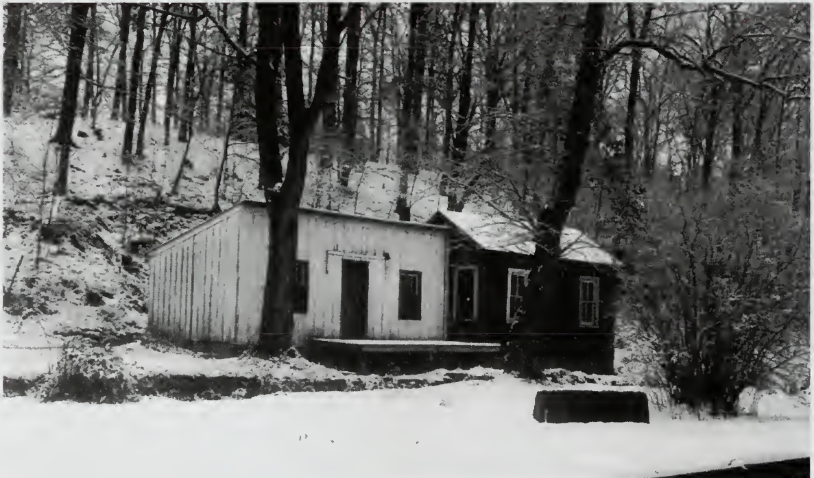
Photograph 32: House at Lock No. 9. This building is a piece-meal structure of uncertain date, hardly usable in its present state, except for the new, shingled addition.
