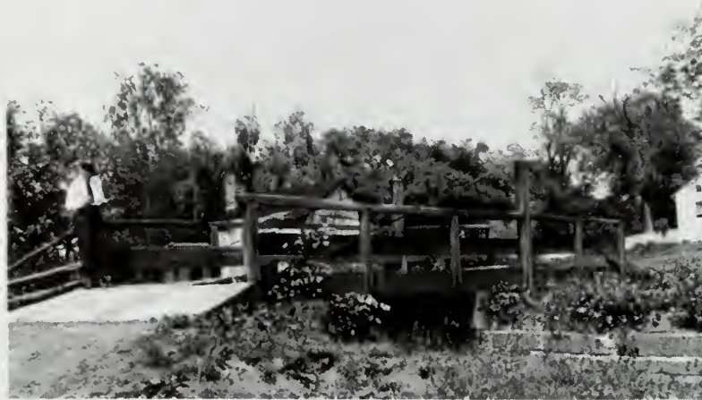
Photograph 6: Swinging Wagon Bridge at Lock No. 25 (Edwards' Ferry). This type of bridge is being used wherever vehicular passage across the Locks is needed.
