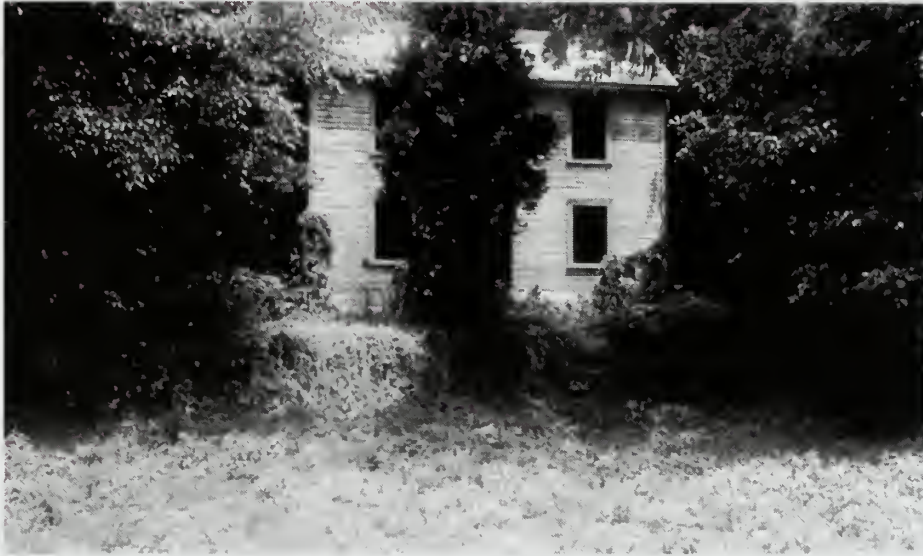
Photograph 41: Frame house at Lock No. 17. In dilapidated state and of unknown date.
