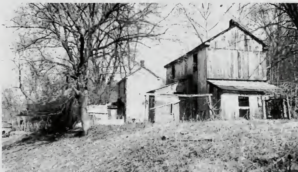
Photograph 50: Frame House No. 2 at Great Falls, from the Canal bank. Some of the material in these buildings will be salvaged for use. The siding from this house will probably be used on the structure at the stop lock above Lock No. 16.
