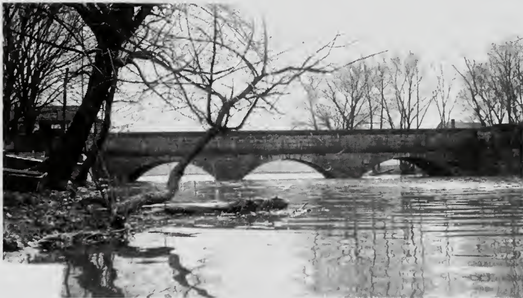
Photograph 15: Seneca Aqueduct, looking from Seneca Creek toward the Potomac. Although this is beyond the present restoration project, it is easily accessible from Lock No 23 and is so handsome and sturdy a structure, typical of such work throughout the length of the canal, that it is illustrated here.
