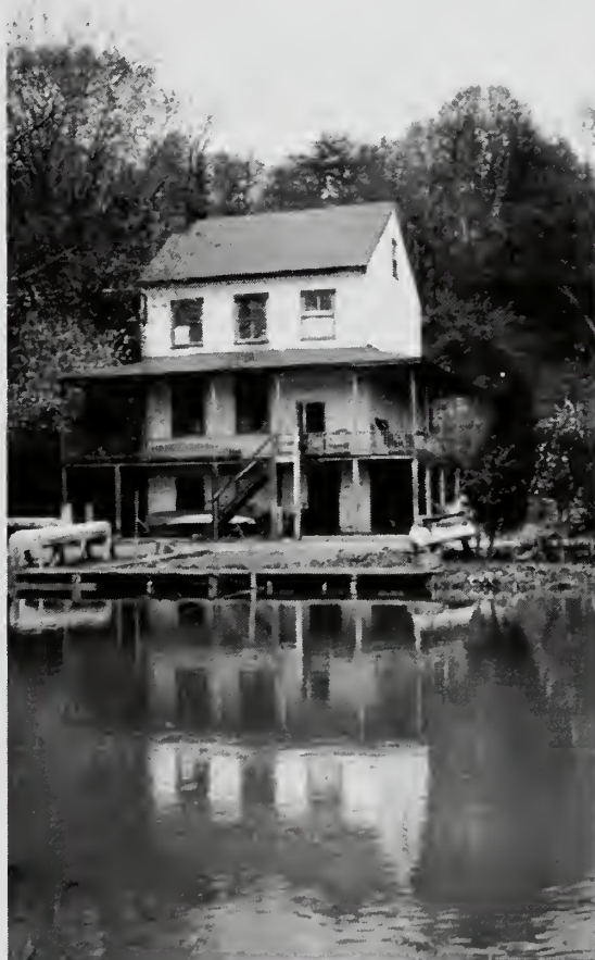
Photograph 11: Fletcher's house from the towpath. This privately owned building is a well known resort for anglers and picnickers. It was built early in the canal period and is of similar architectural character to the canal houses.
