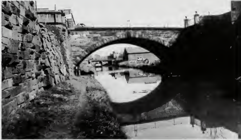
Photograph 4: Wisconsin Avenue Bridge, looking east along towpath.
