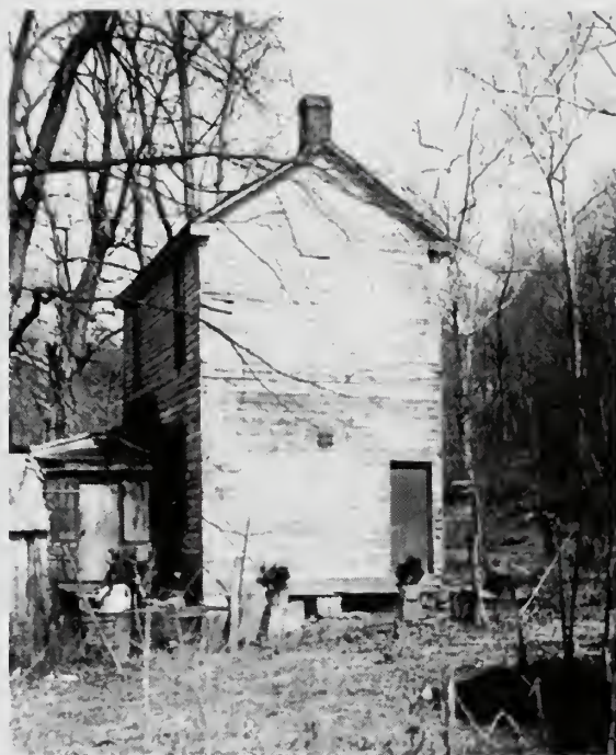
Photograph 49: Frame House No. 1 at Great Falls. This will probably be demolished.
