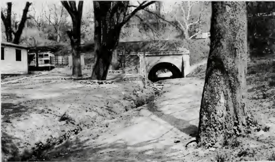
Photograph 10: South Arch, Fletcher's underpass.
