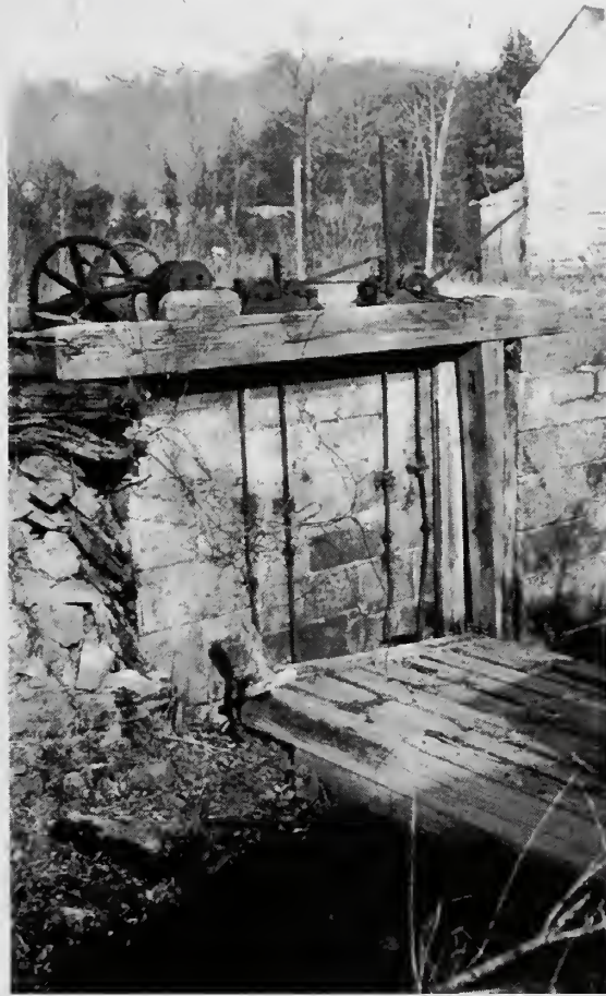
Photograph 2: Drop gate and machinery at Lock No. 12. Gate in open position.
