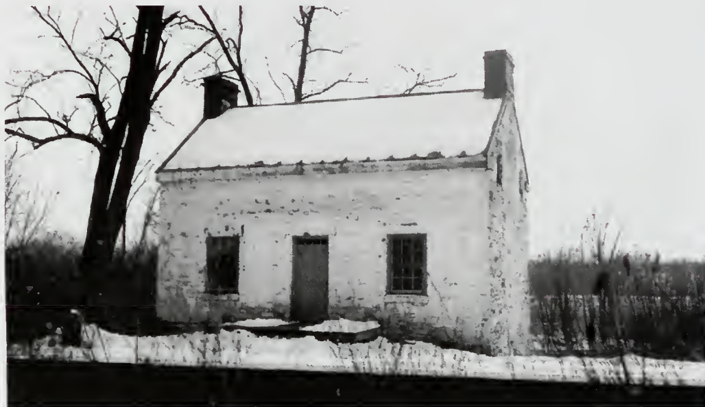
Photograph 53: House at Lock No. 22, with Lock wall in foreground. These chimneys vary from type in being built of cut Seneca sandstone instead of brick. The trees here are black walnut.
