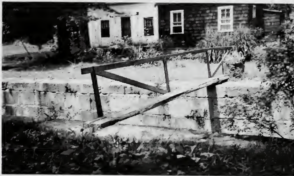
Photograph 7: Footbridge across Lock No. 9.
