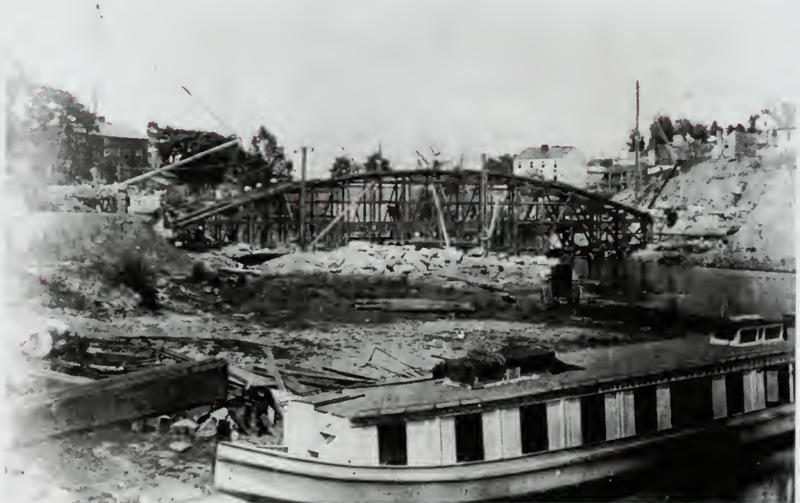
Photograph 60: Cumberland Packet lying at Lock No. 1, Georgetown. In the background appears the centering for the masonry arch of the Pennsylvania Avenue Bridge.
