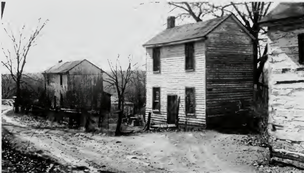
Photograph 48: A corner of the Log House in foreground and beyond it frame Houses No. 1 and 2, built about the same time. They are of little value and will probably be demolished and the material salvaged for use elsewhere on the canal.
