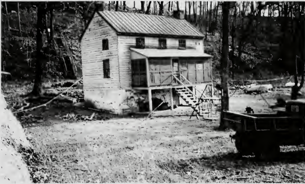
Photograph 24: The house at Lock No. 5, a frame building on masonry walls. This is being restored for use, with the addition of dormers for added light and ventilation, and of plumbing.
