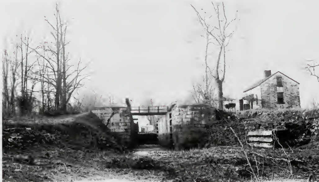
Photograph 37: House at Lock No. 13 shown in relation to the Lock. As both gates are open, Lock No. 14 can be seen in the background. The house is in usable condition and continues to serve.
