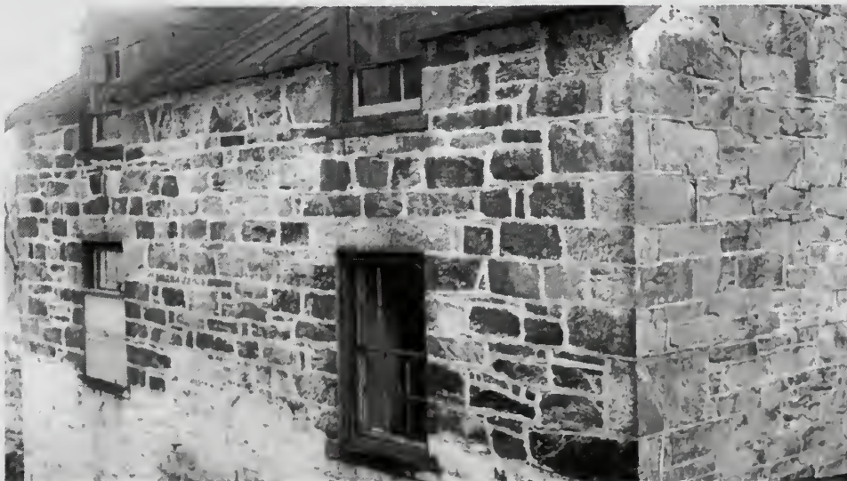
Photograph 40: The substantial character of the masonry is clearly seen in this picture, as well as the type of dormer windows.
