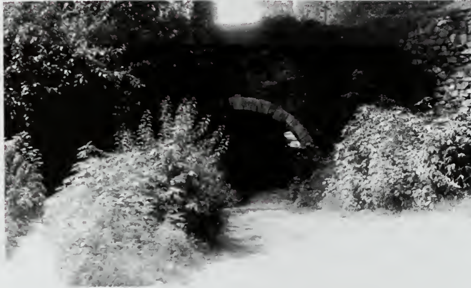
Photograph 8: Foundry Branch Underpass, South Arch.
