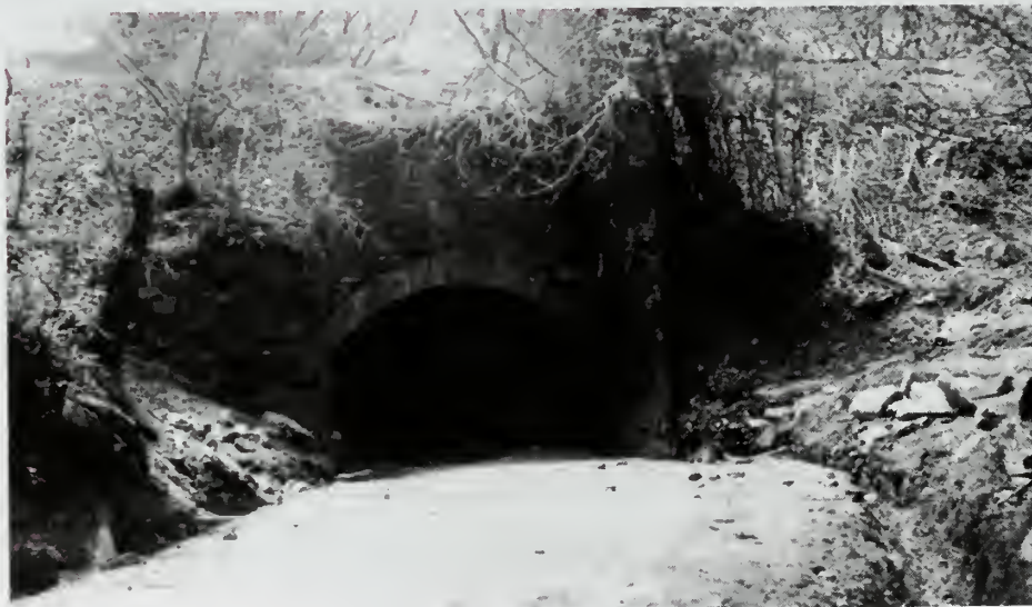
Photograph 9: North Arch, Fletcher's Underpass.
