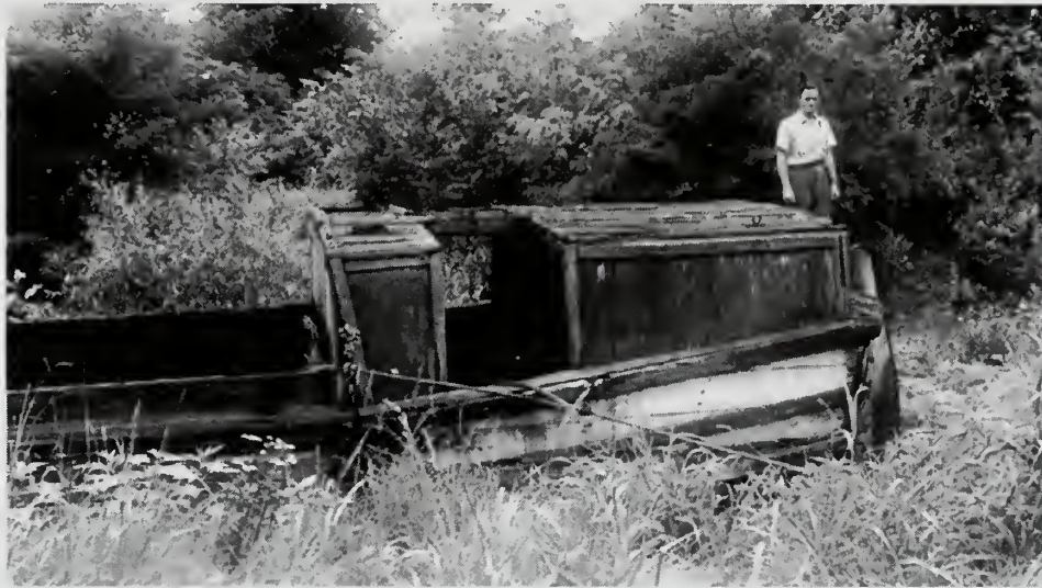
Photograph 57: Bow of canal barge No. 57 at Hancock, Maryland, showing the mule stable.
