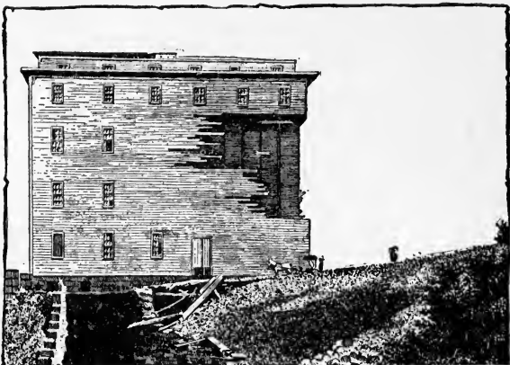
FIG. 9.—Showing effect of expansion of air contained in a hollow wall during the passage of the storm.
