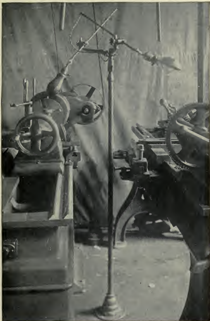
Plate VIII: To eliminate swinging wires and shades, this simple gas pipe fixture is used in the Washburn Shops of the Worcester Polytechnic Institute. Wiring is beneath the floors (See chapter X)
