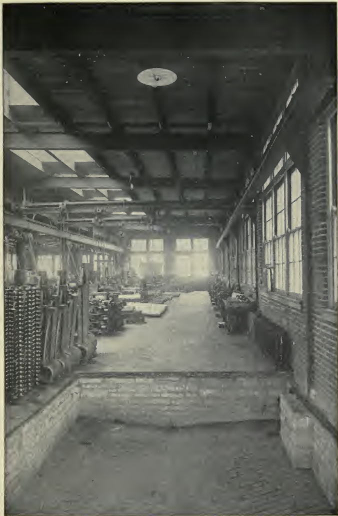
Plate XV: To save coal in winter the shipping platform is built inside the building so that a sliding steel curtain will enclose it. (See chapter XIII)
