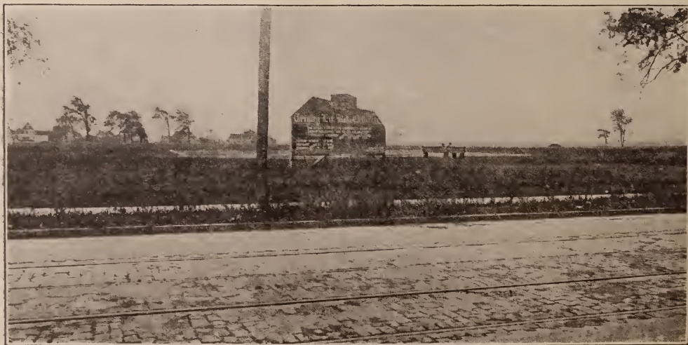
FIRST STEP IN CHURCH BUILDING—SECURING THE SITE
