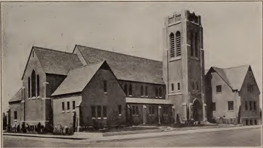
FIRST REFORMED CHURCH, LOS ANGELES, CALIFORNIA,
