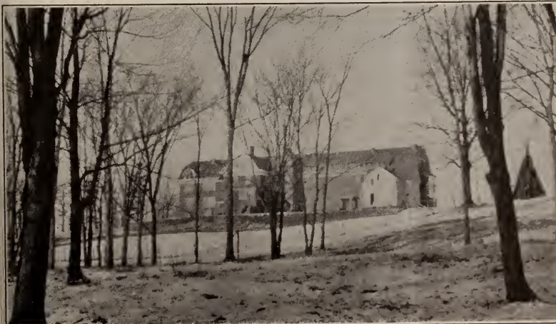
REAR OF INDIAN SCHOOL BUILDING, NEILLSVILLE, WIS.
