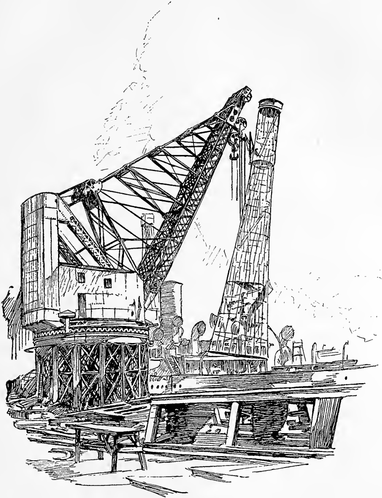
HOISTING A BATTLESHIP TOWER WITH WIRE ROPE
