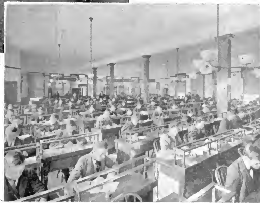
Putnam, Photo. Partial view of Main Study Hall. Union Eng Co.
