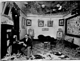
Interior of Reception Room. Taken by Flashlight.
