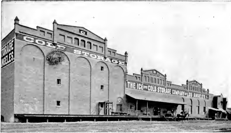
THE ICE AND COLD STORAGE PLANT, 7TH AND S. F. RY. TRACKS.
