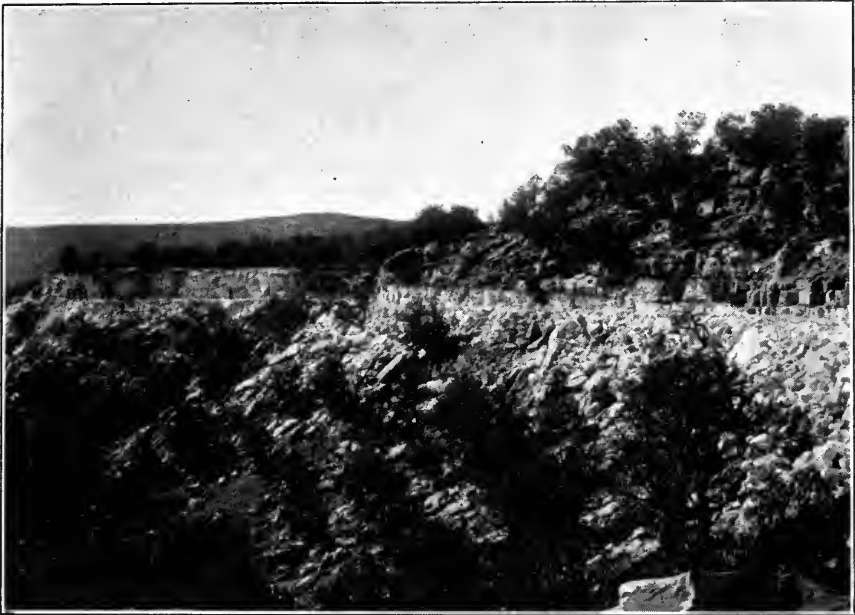
ROCK-CUT ON LINE OF CANAL.
