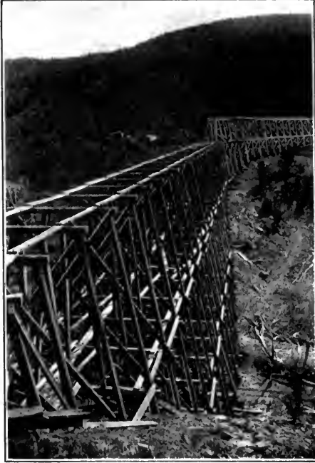
TRESTLE ACROSS THE CAÑON.
