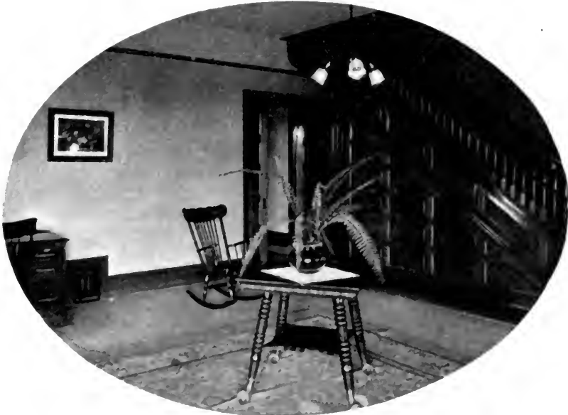
RECEPTION ROOM, FULLERTON HOSPITAL.
