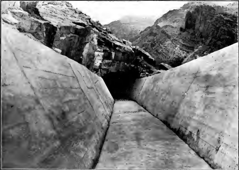
A TUNNEL ON THE POWER CANAL.
