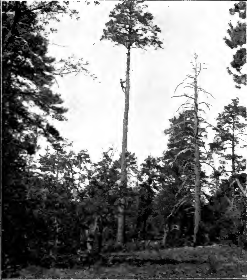
TRIMMING THE SPAR TREE FOR STEAM LOG SKIDDER
