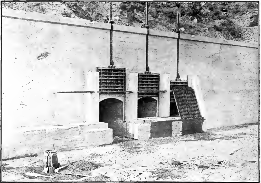
GATES AT INTAKE OF POWER CANAL.
