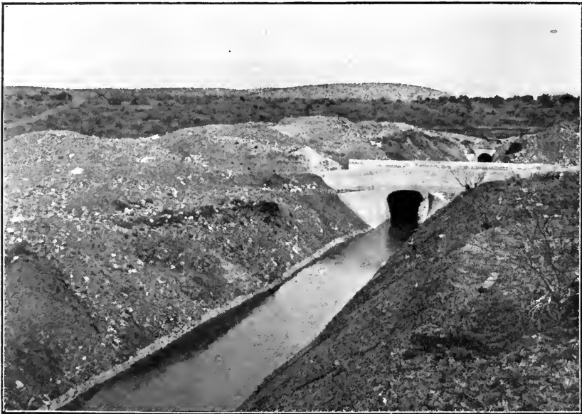
ON THE POWER CANAL
