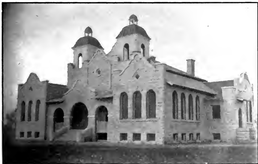
The Porterville High School Built from granite quarried within two miles of Poterville
