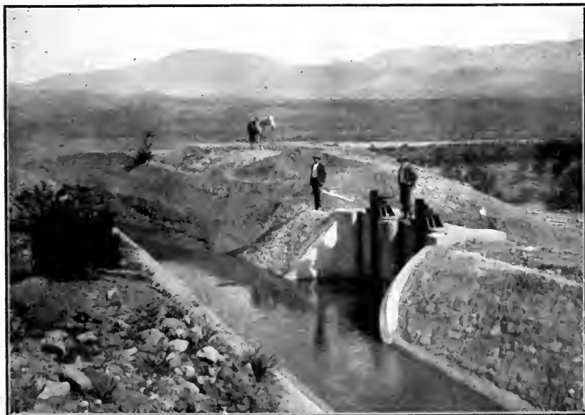
SLUICE GATES ON POWER CANAL.
