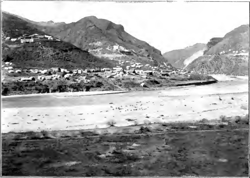
TOWN OF ROOSEVELT, U. S. R. S. HEADQUARTERS, CEMENT MILL, ETC.
