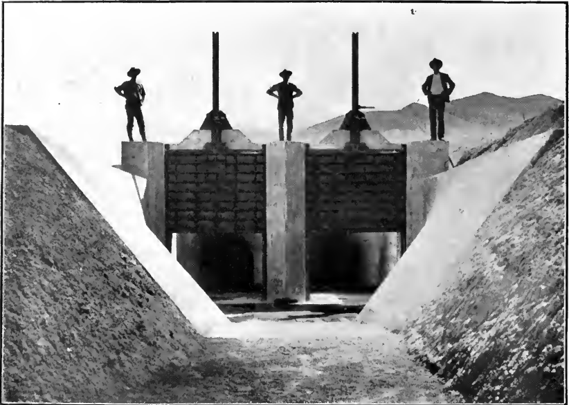
EXIT END OF COTTONWOOD PRESSURE PIPE.
