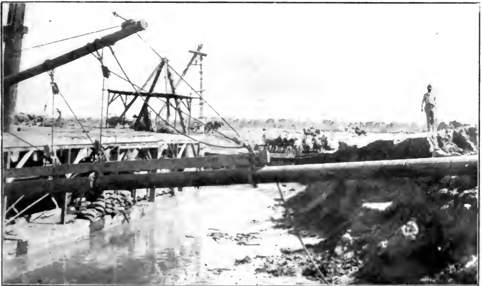
SUCTION DREDGE AND SCRAPER TEAMS CUTTING CANAL TO WOODEN HEADGATE.
