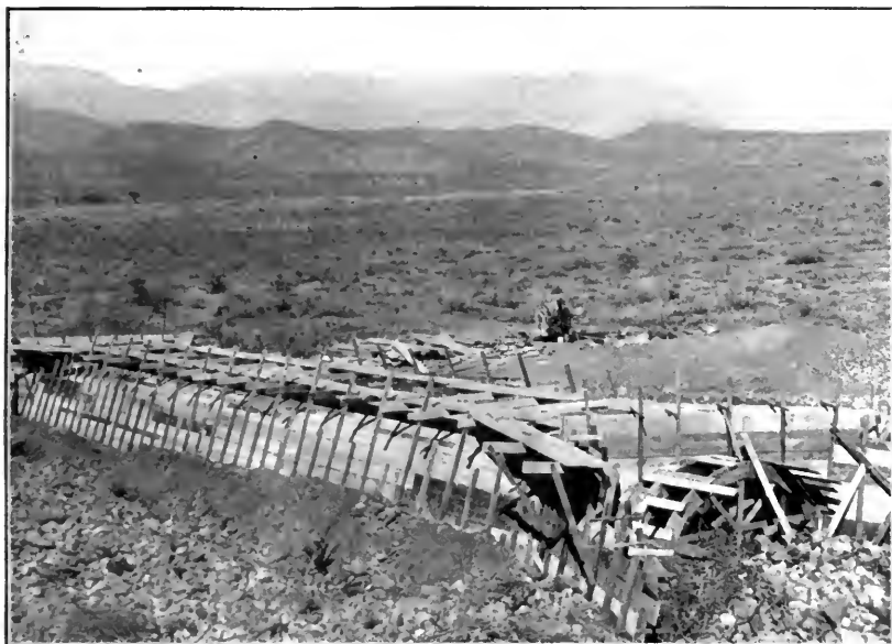
FORM FOR CONCRETE CULVERTS USED ON POWER CANAL AT TONTO.
