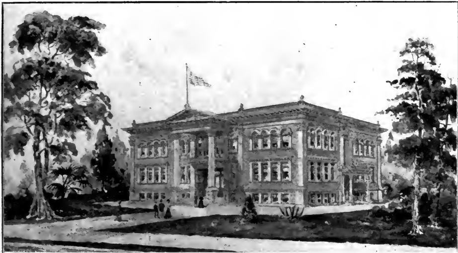
SAN FERNANDO HIGH SCHOOL--IN COURSE OF ERECTION
