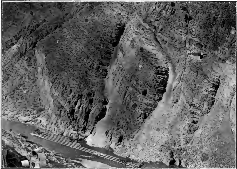
LOOKING DOWN ON THE TONTO DAM SITE.
