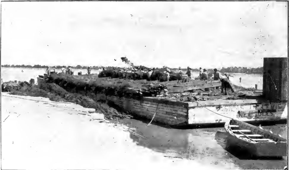
MAKING BRUSH MATS ON THE BARGE
