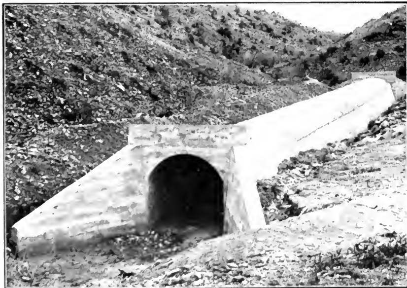
CONCRETE PIPE CULVERT.
