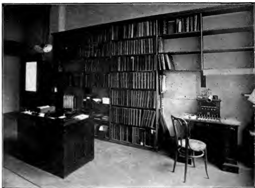
PUBLIC WAITING ROOM, CLERK'S OFFICE AND TELEPHONE EXCHANGE
