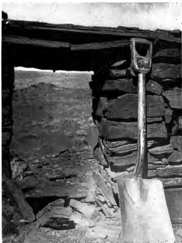
" WHERE ONCE WERE DOORS AND WINDOWS "
