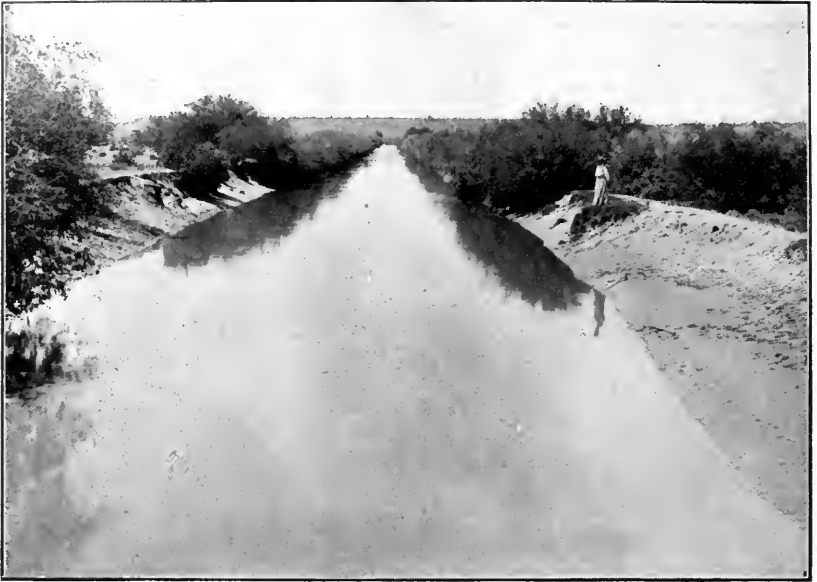
CANAL NEAR PHOENIX.
