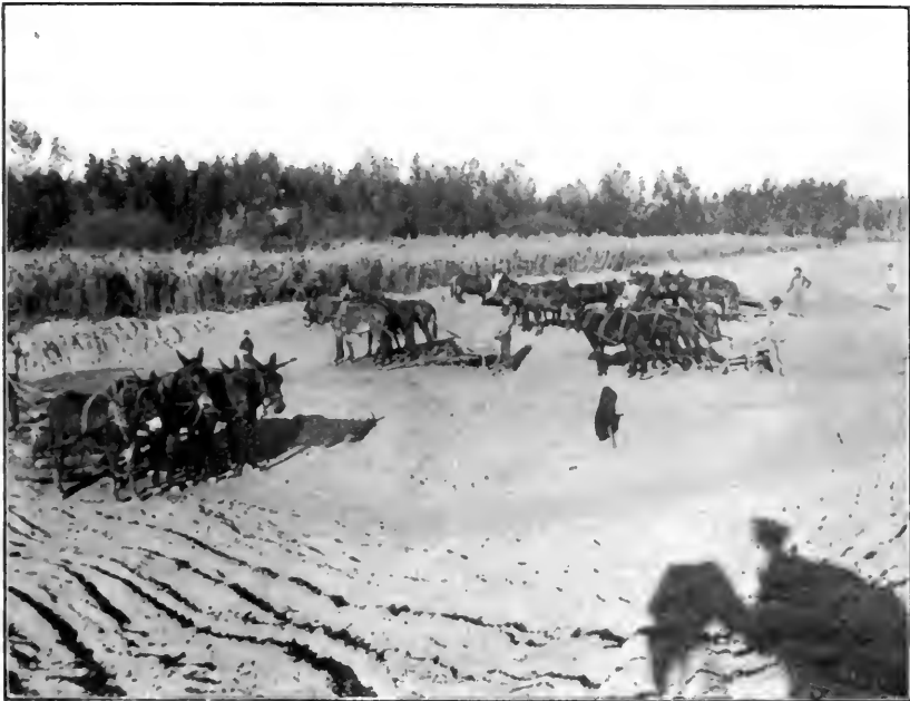
BUILDING LEVEES ON THE COLORADO RIVER NEAR YUMA
