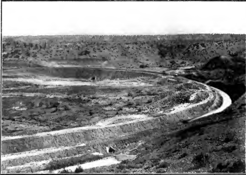
COMPLETED SECTION OF POWER CANAL.
