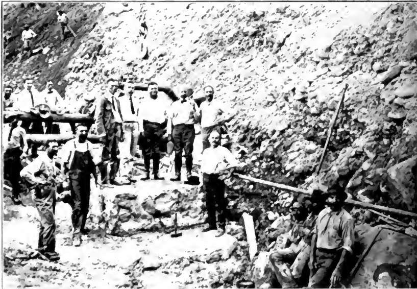
FIRST STONE IN ROOSEVELT DAM SITE, SEPTEMBER 20, 1906
