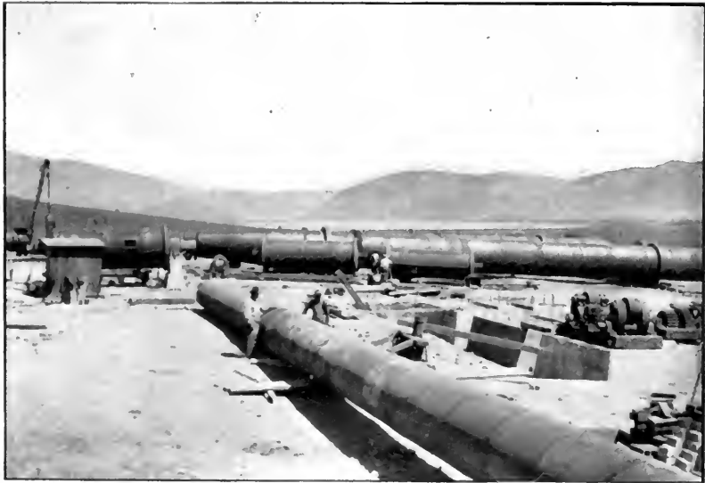
A BIT OF AQUEDUCT WORK
