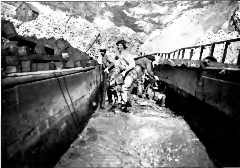
CLEANING UP THE BLOCKS IN THE SLUICE-BOXES AT LA GRANGE
