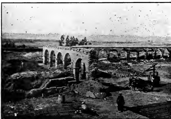
Rebuilding Corridors at San Luis Rey Mission
