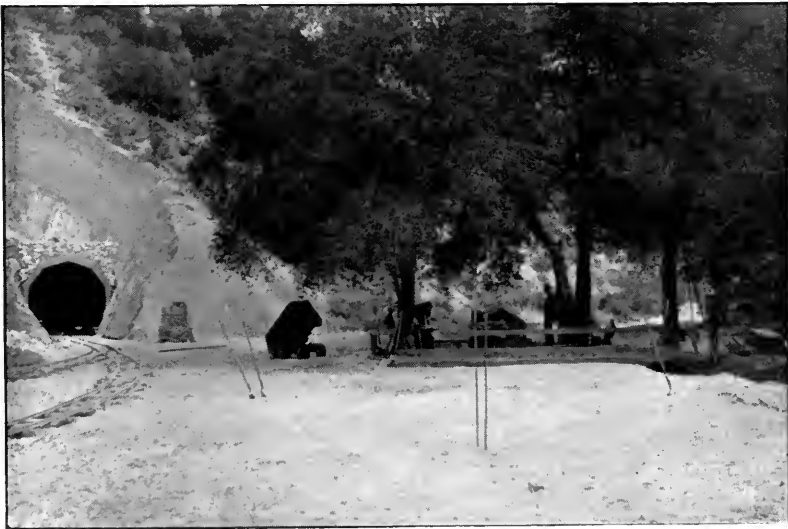
SOUTH PORTAL ELIZABETH LAKE TUNNEL
