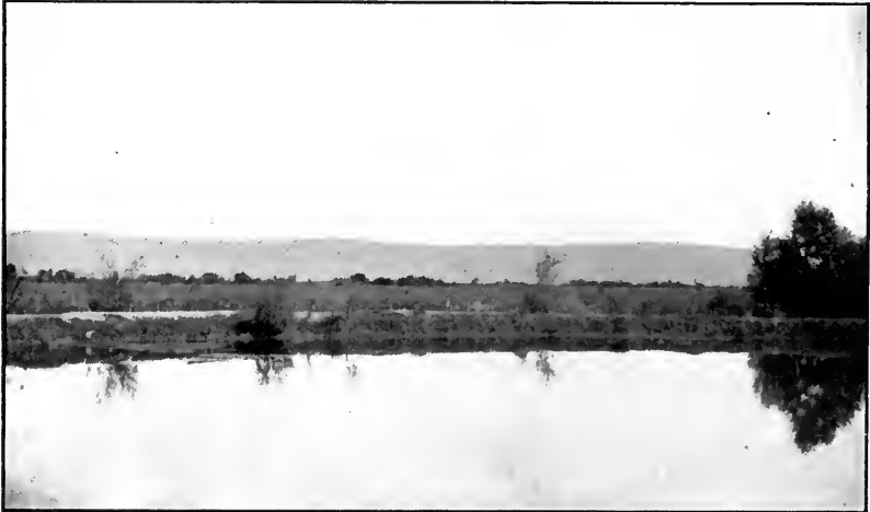
A RESERVOIR ON THE TORRES RESERVATION
