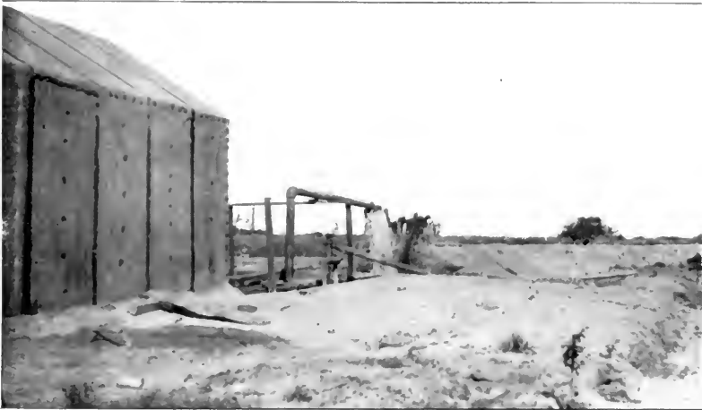
PUMPING PLANT AT COACHELLA
