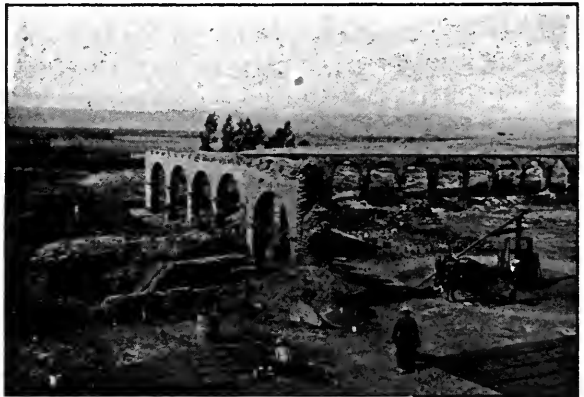
Rebuilding Corridors at San Luis Rey Mission
