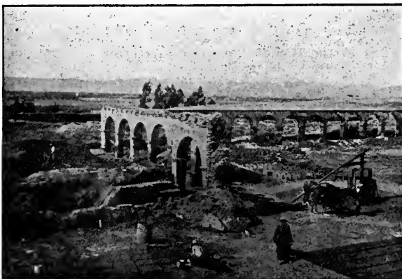
Rebuilding Corridors at San Luis Rey Mission
