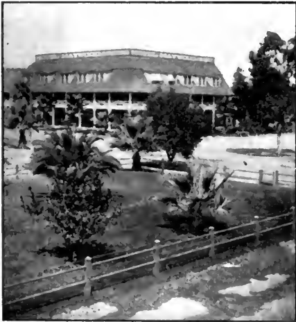
Hotel Maywood, Corning, Cal.
