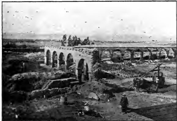
Rebuilding Corridors at San Luis Rey Mission
