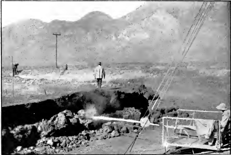
HYDRAULIC DREDGE AT WORK IN THE OWENS VALLEY
