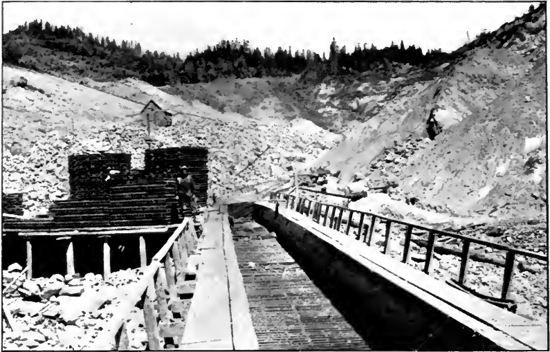
STEEL-RAILS USED AS RIFFLES AT LA GRANGE MINE
