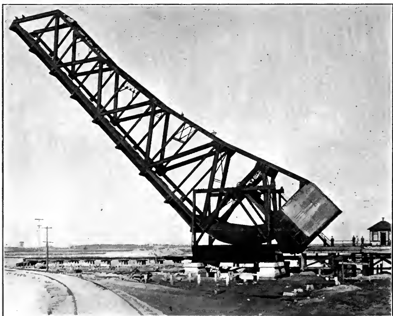
BASCULE BRIDGE RAISED, SAN PEDRO
