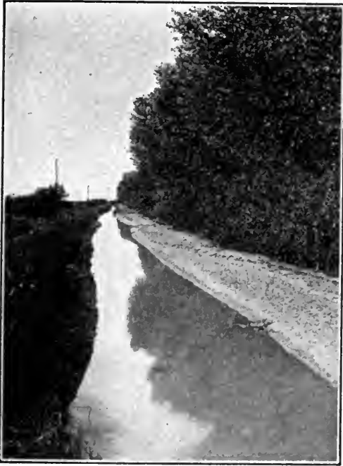
IRRIGATION CANAL, CALEXICO
