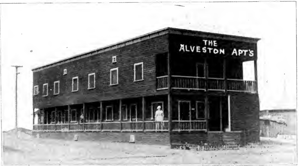
A Typical Balboa Modern Apartment House
