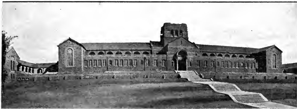
Polytechnic High School, covering 13 acres, cost $350,000, Roman Architecture, Santa Monica.
