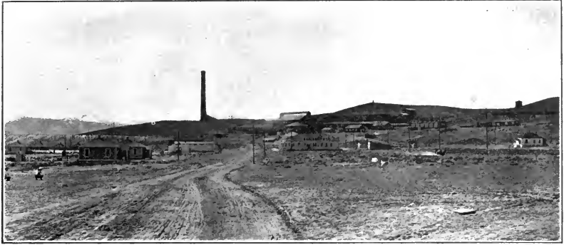
DISTANT VIEW OF THE MASON VALLEY SMELTER, CAPACITY 2,000 TONS DAILY, THOMPSON, NEVADA.
