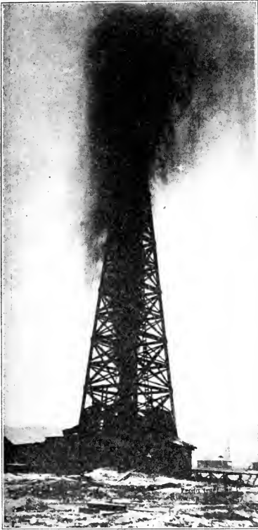
Pacific Crude No. 1, gushing 15,000 bbls. of oil daily, before it caught fire.
