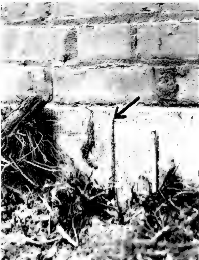
Fig. 6.—Termite tube built up on the outside of the concrete foundation of a house. This tube is small and rather difficult to detect. The foundation must be carefully examined to locate such inconspicuous tubes.
