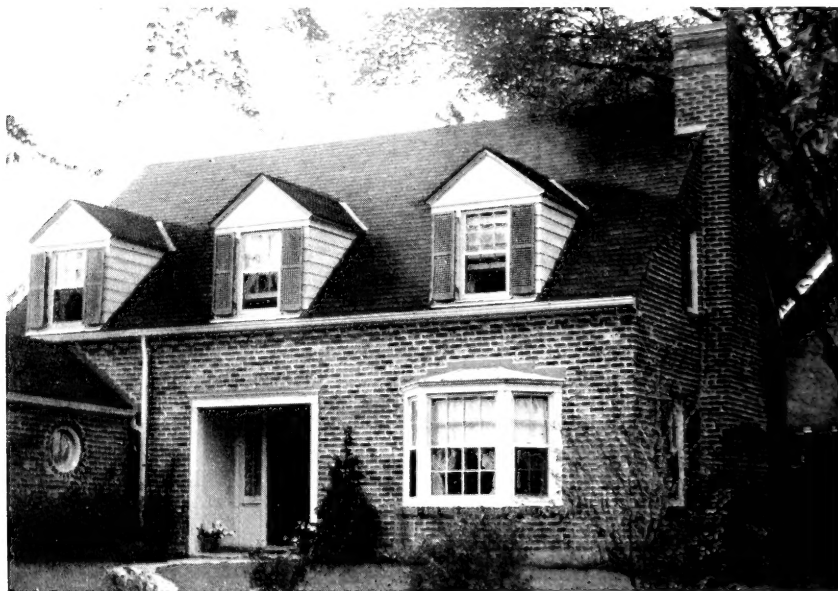
The home that is built to discourage termite attack saves its owner worry, time and money.
