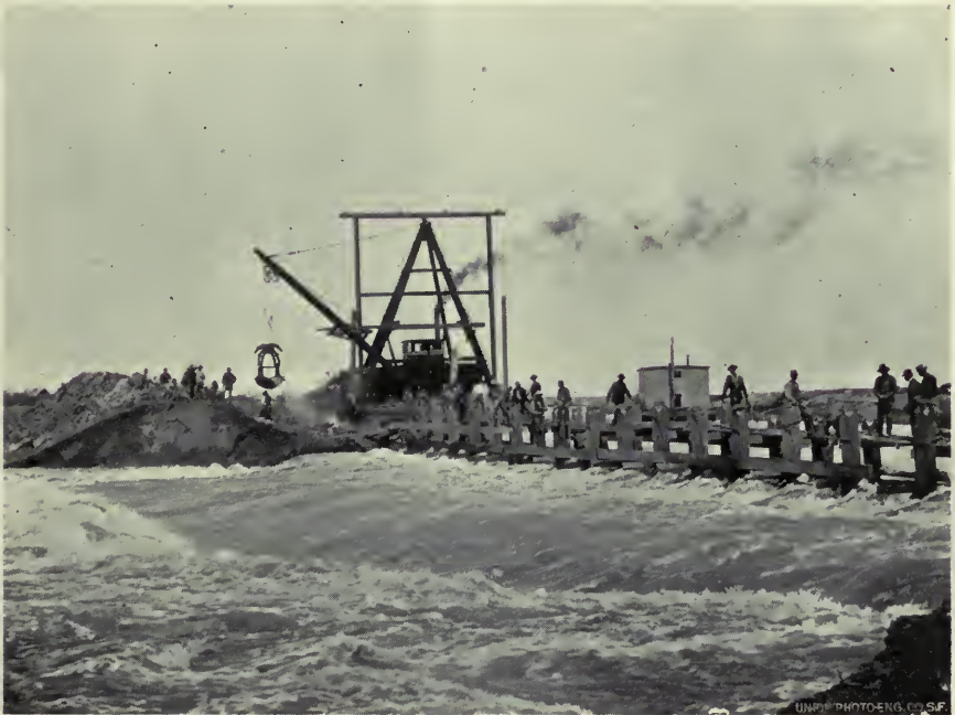
REPAIRING A BREAK.—CLAMSHELL DREDGE.
