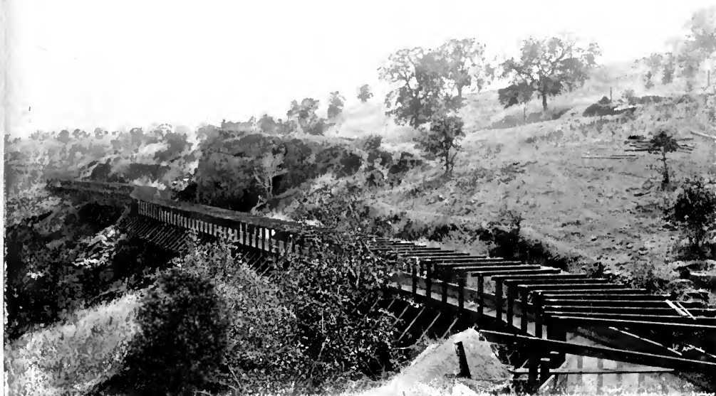
FLUME THREE, 2350 FEET LONG.
