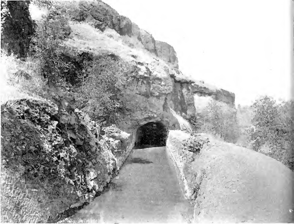
LOWER END OF TUNNEL TWO, 1037 FEET LONG:
