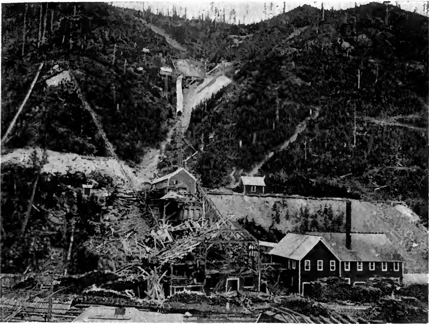
FRISCO MILL AFTER THE EXPLOSION.
