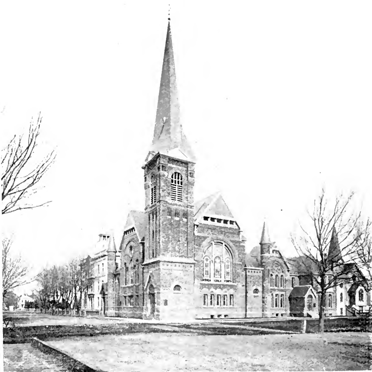
CENTRAL METHODIST EPISCOPAL CHURCH
