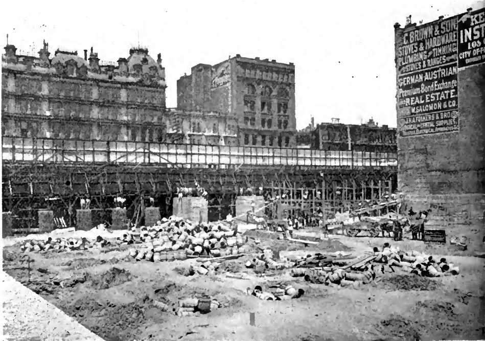
THE CONCRETE PIERS, BUILT BY GOODMAN.
