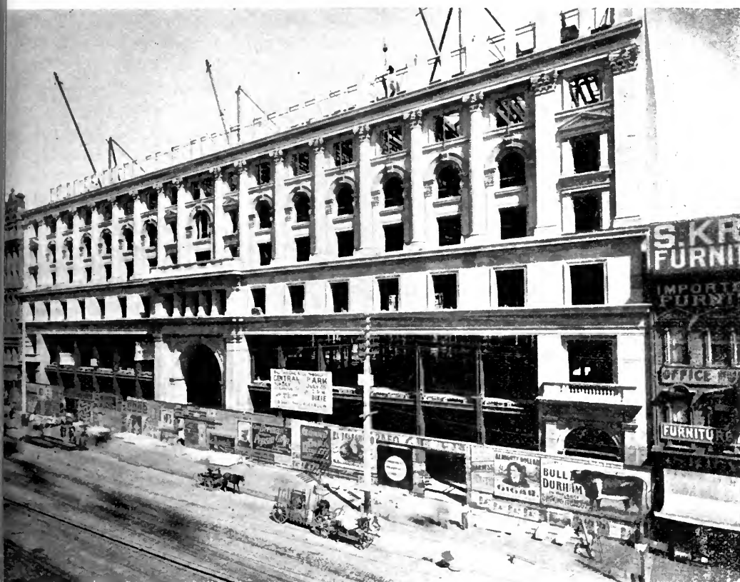
BUILDING UP THE STONE FRONT. J. D. MCGILVRAY, BUILDER.
