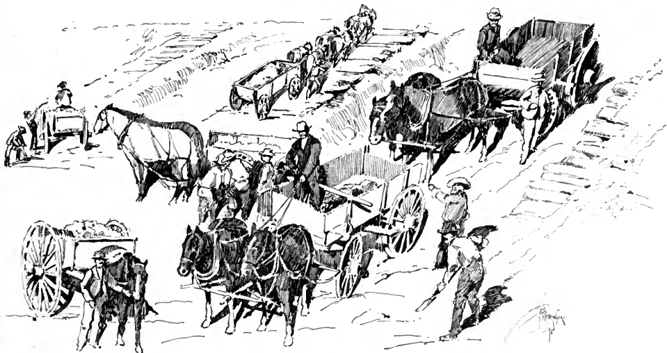
BUCKMAN'S TEAMS EXCAVATING FOUNDATION.
