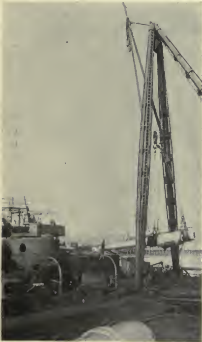
Installing a 13-inch gun on board the Oregon at the Union Iron Works.
