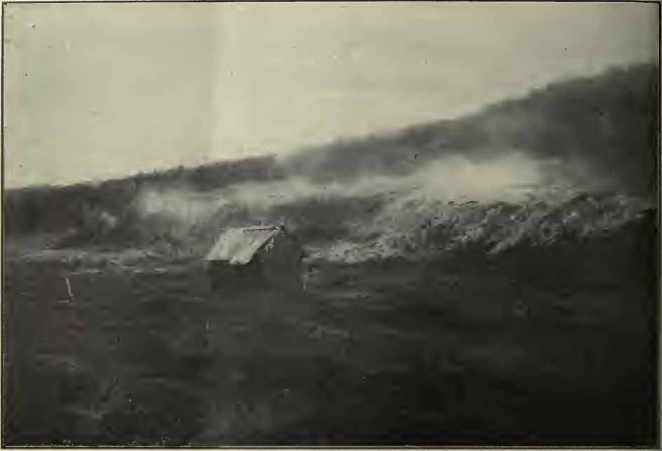
The sulphur banks and bath house on the bank.
