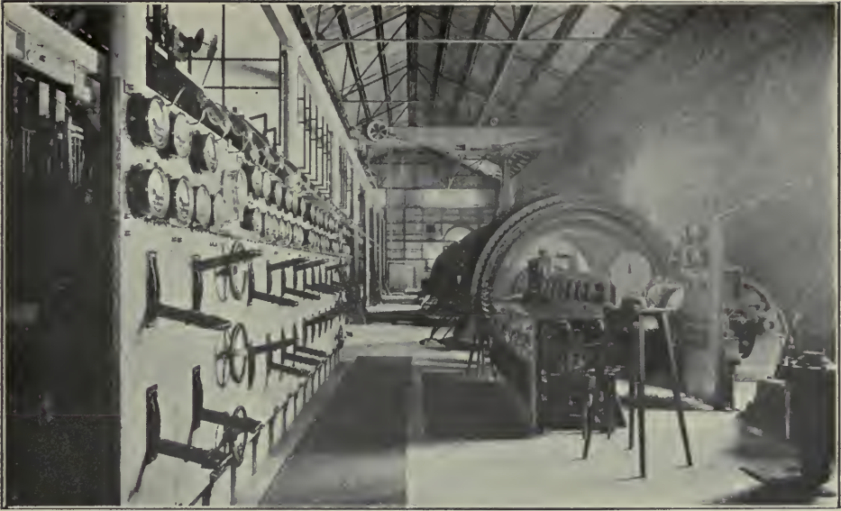
Showing switchboard, operating table, and 2,000 Kilowatt generators.
