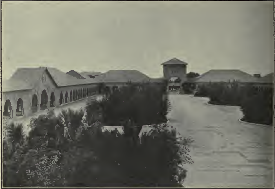
General View of the Inner Quadrangle.
