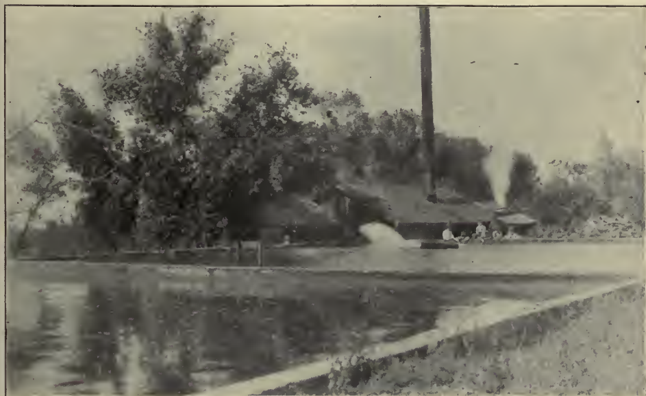
Pumping plant near Davisville.
