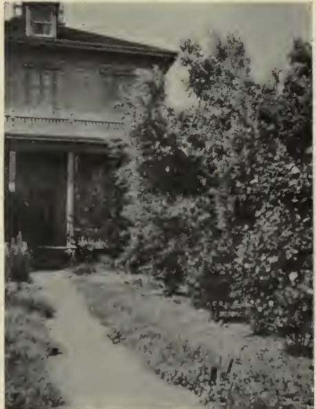
Supervisor Decker's home at Dunningan.
