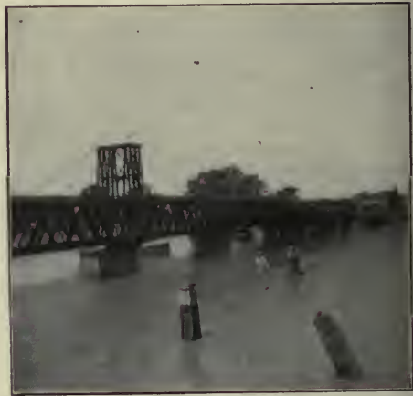
Steel bridge connecting Yolo and Sacramento Counties, between Broderick and Sacramento.
