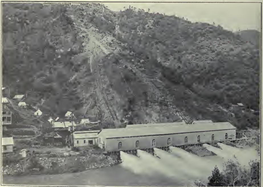
Colgate Power House, - Pipe lines, Pinstock, and a section of flume.
