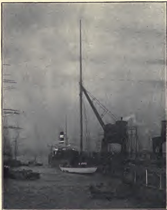
Setting the mast.
