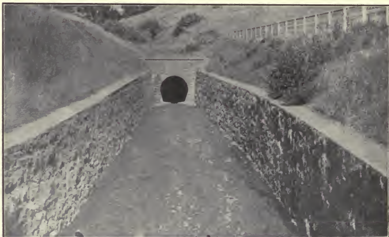
Waste-way and tunnel number three
