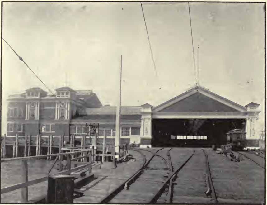
View showing entrance for electric car from long trestle
