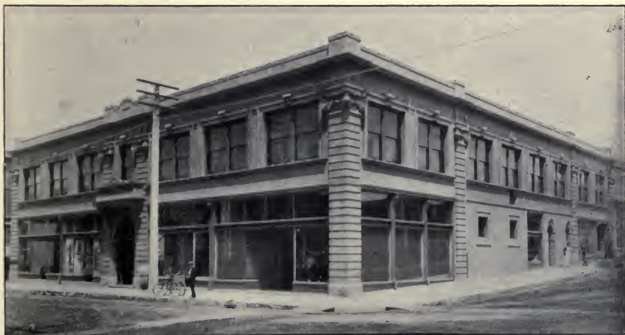
View of Gross Building, Eureka, Humboldt Co., Cal.
