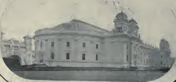
Oriental Exhibits Building.
