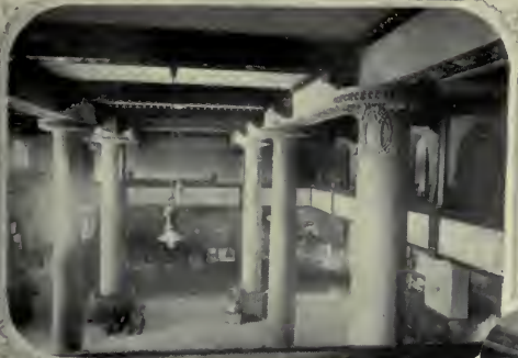
VIEW OF OFFICE FROM PARLOR FLOOR MEZZONINE
