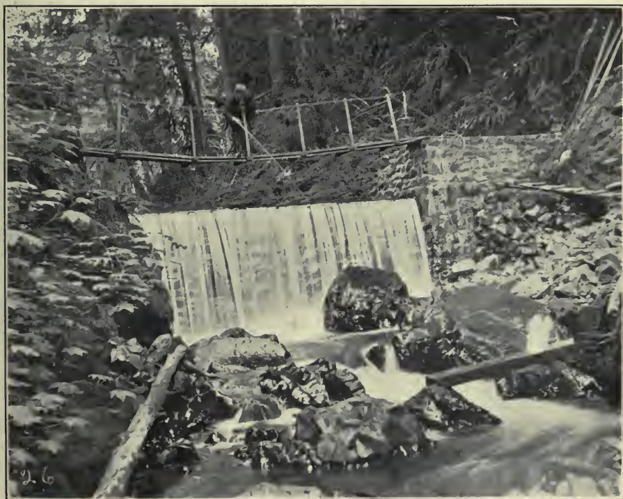
Astoria water supply—headgate.
