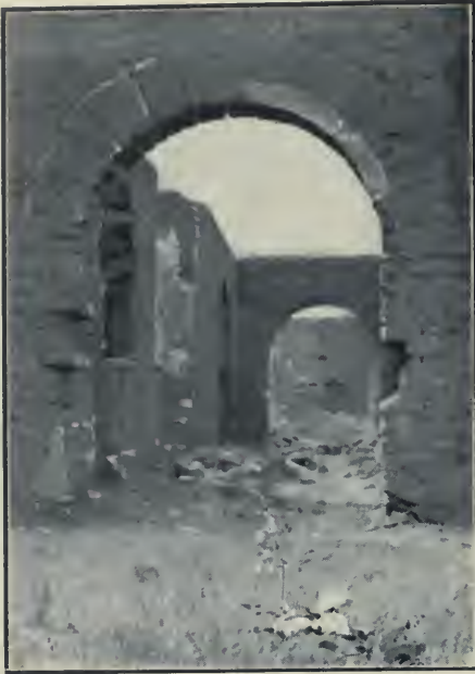
Crumbling walls of Fort Lowell.
