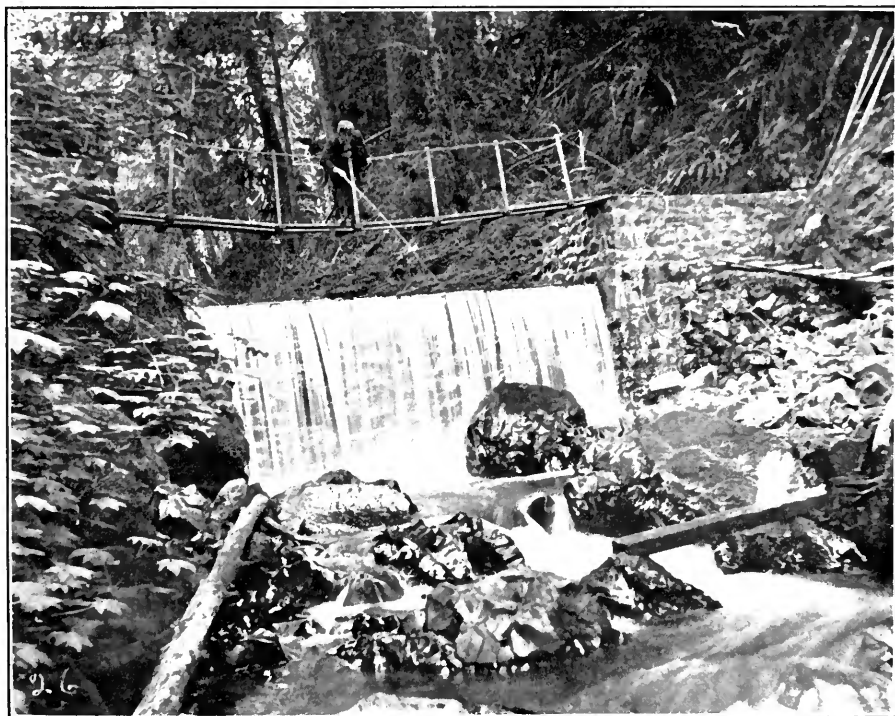
Astoria water supply—headgate.
