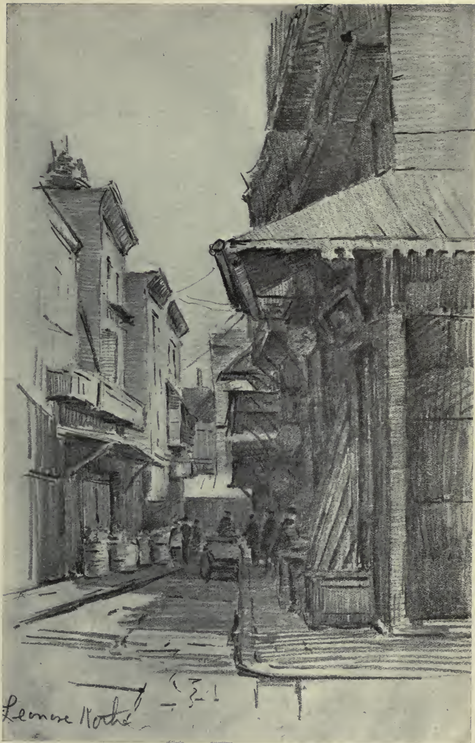
Fish Alley, seen from Washington Street. (3-1)
