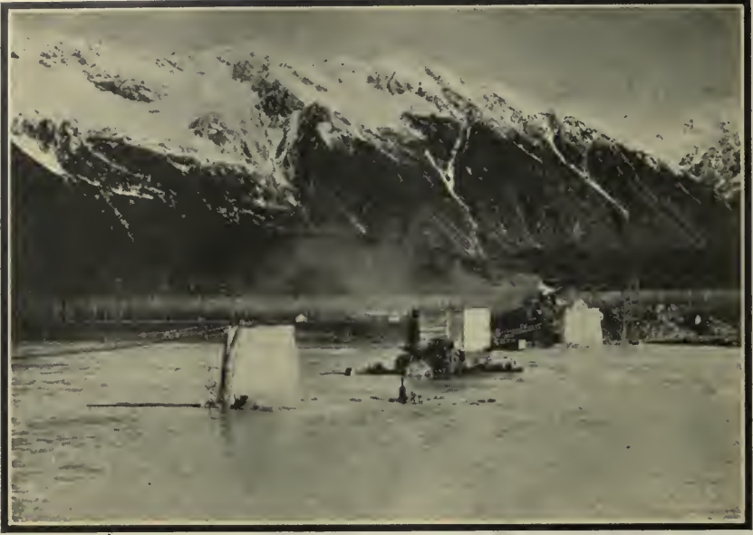
Concrete piers for the Miles Glacier bridge across the Copper River, made strong enough to withstand great ice pressure.
