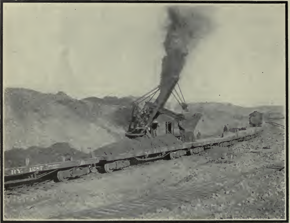
Loading dredge tailings on cars for use as railroad ballast.
