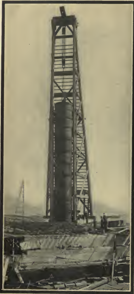
Driving one of the 60-foot caissons which support the wharf.
