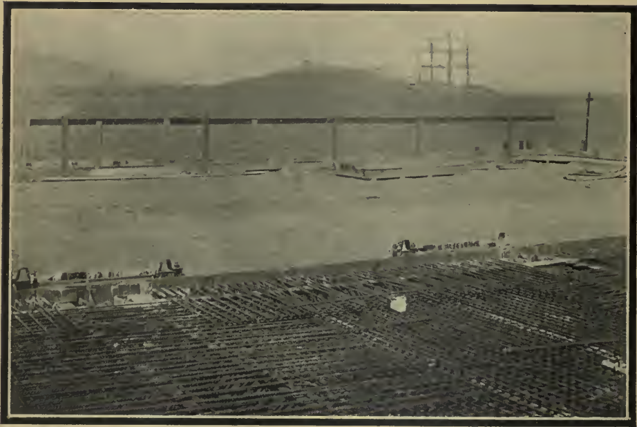
Wharf floor, showing reinforced steel construction.
