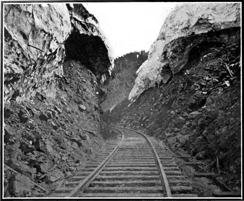
August remains of a snow slide on the Alaska Northwestern Railroad on Teni peninsula.
