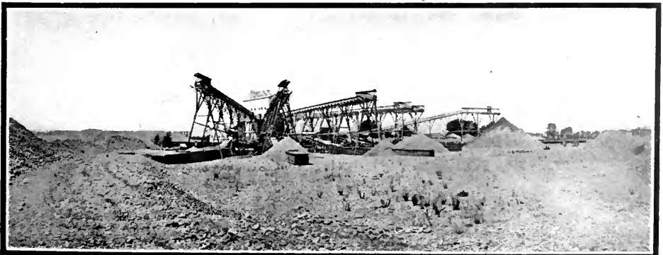
Rock dredging plant utilizing dredge tailings.
