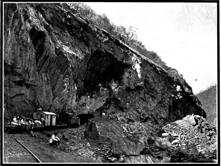
On line of new railroad.
