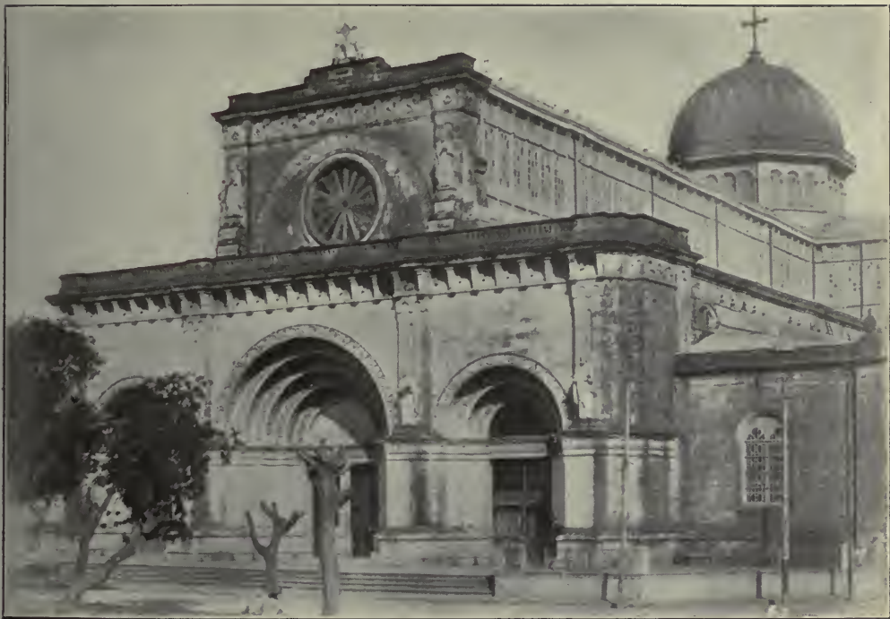
The Plaza McKinley, entrance to the Catholic Cathedral, Manila.
