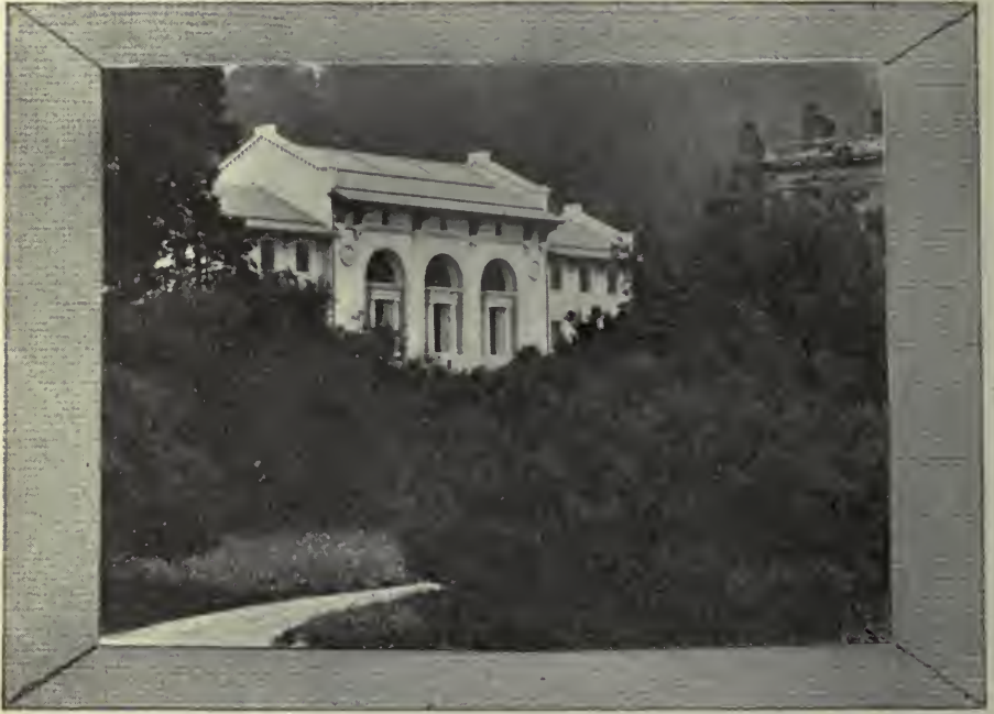
Mining Building, University of California.
