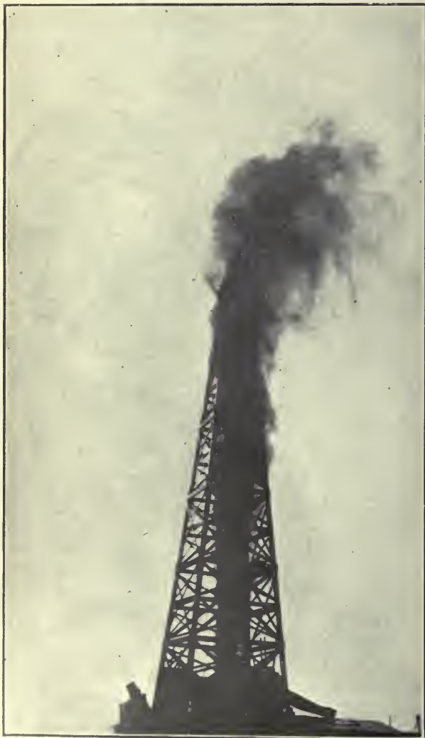
Photo taken a few days before the well caught fire. This view shows the oil stream breaking from control and shooting upwards in a spray far above the top of the derrick.
