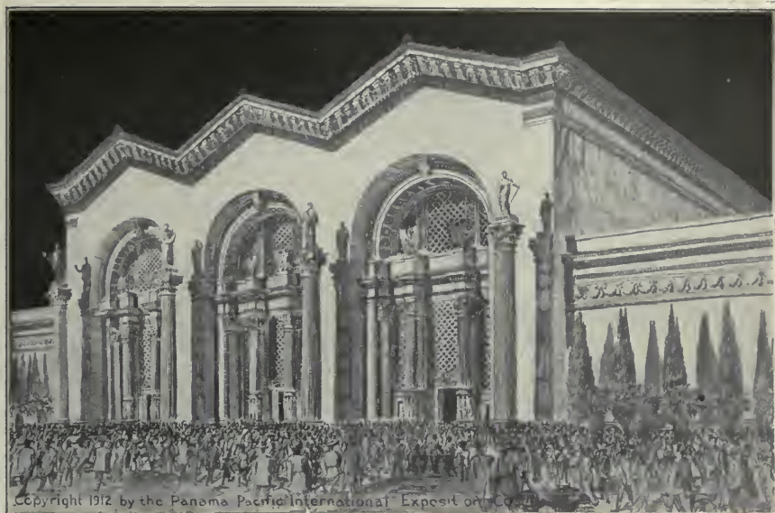
Facade of the Machinery Palace just completed and accepted by the Exposition Company.
