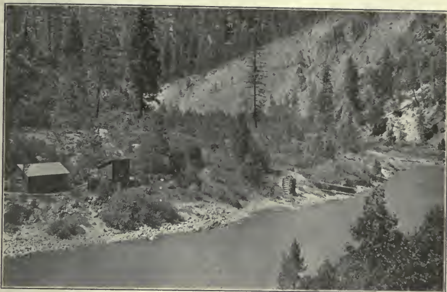
The two shacks built by the brother, sister and cousin beside the old river channel, which had produced great riches in placer mining.
