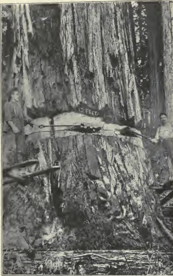
Tree cutters preparing to fall a big redwood twelve feet across the cut.
