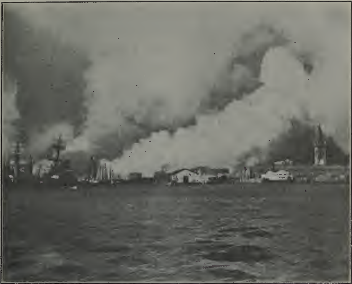
A SECTION of the big fire of April, 1906, advancing on the ferry system depots of San Francisco.
