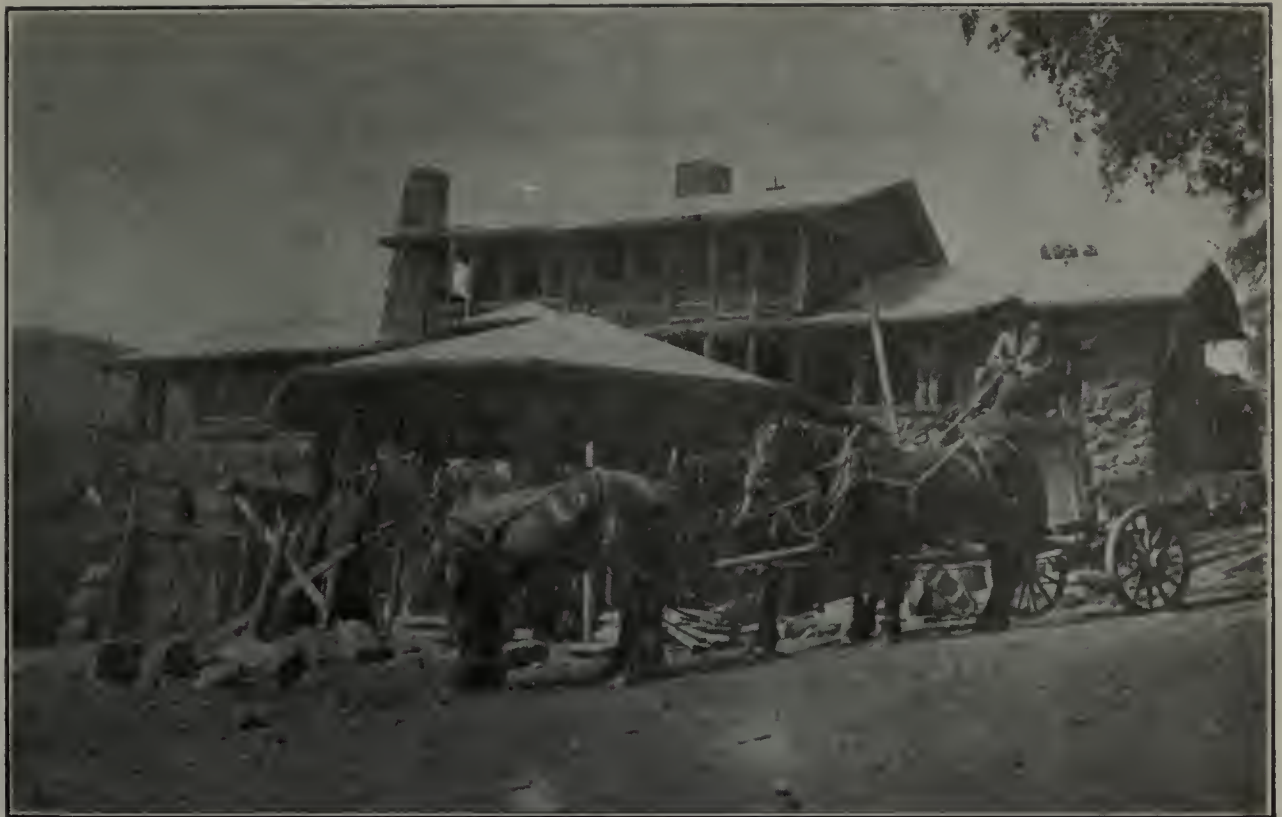
“Wolf House” before the destructive fire.
