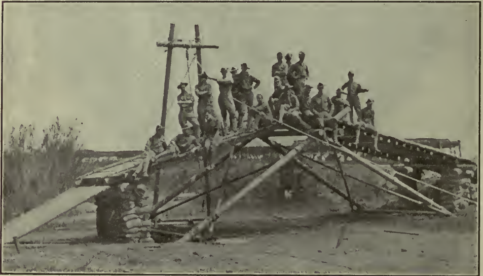
U. S. Marine officers being schooled in bridge construction.
