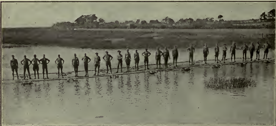
U. S. Marine officers' school and advance base, Port Royal, S. C., demonstrating construction of foot pontoon bridges made of bamboo and ordinary kegs.
