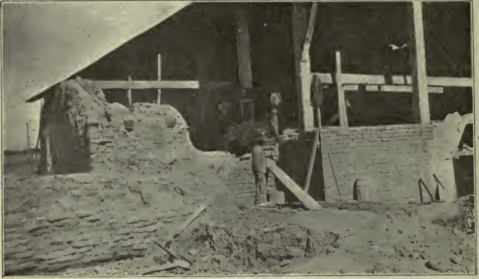
The Western Wall of the Church.—“The main entrance where many a peon laborer, with typical languor, was working on the wall which, weakened by numerous treasure-seeking excavations, had recently given away, crushing with it a part of the Baptistry room.
