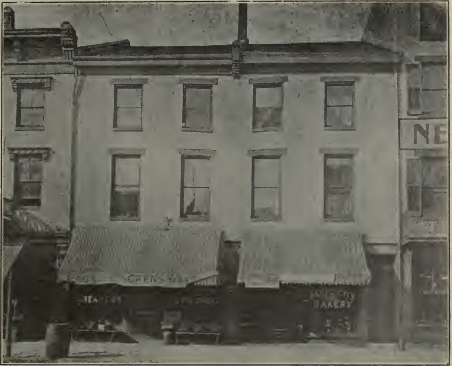
Publication office of the Hannibal Union. In the second story Mark Twain worked as a printer. —From a recent photo of the building.
