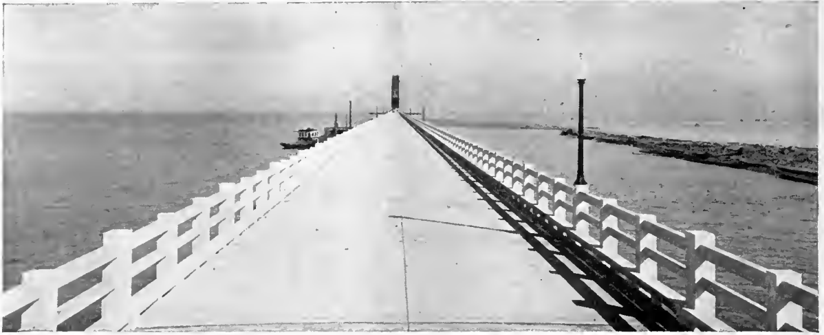
San Francisco Bay Bridge—"The Bridge the Oyster Built"
