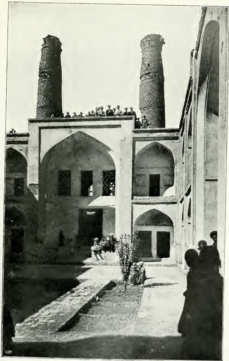
182. TWO OLD TOWERS IN TEBBES.
