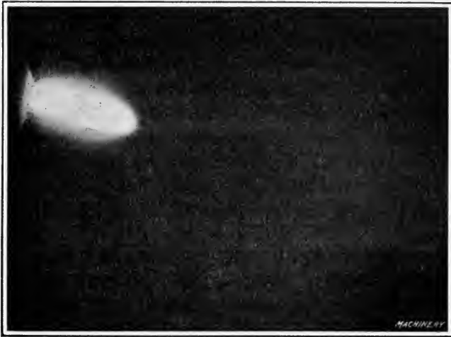
Fig. 2. Neutral Flame photographed through a Light Filter
