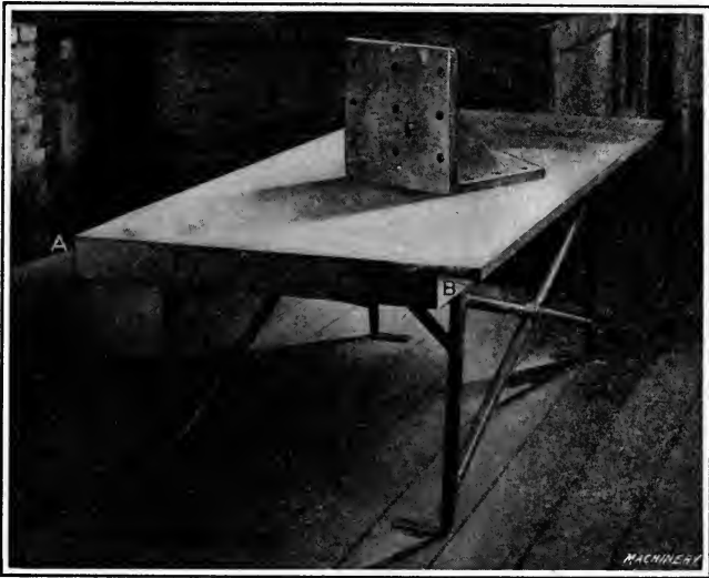
Fig. 23. Another View of Welding Table and Angle-plate
