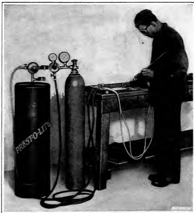
Fig. 6. Complete Lead-burning Outfit in which Air and Acetylene are used
