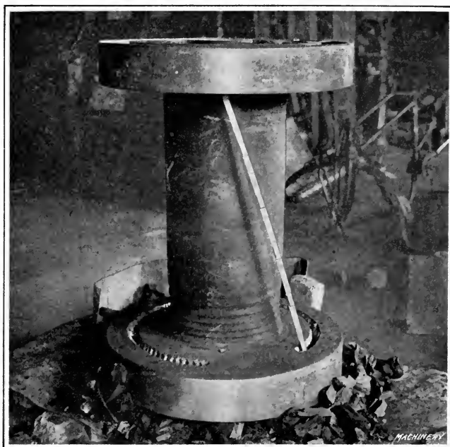
Fig. 7. Hoisting Engine Drum prepared for Welding
