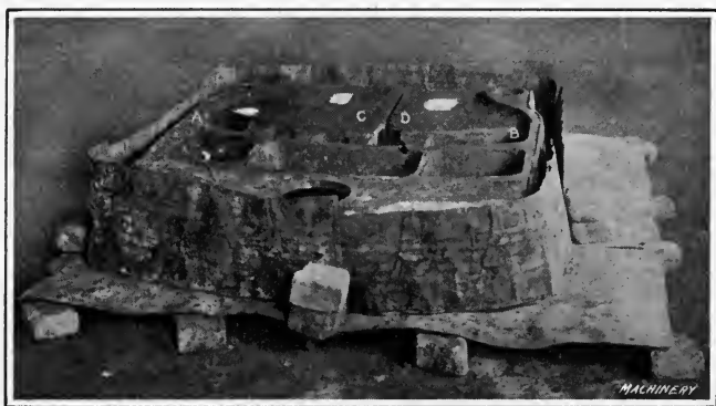
Fig. 40. Heating Boiler Casting ready for Preheating Fire to be started
