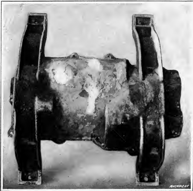
Fig. 17. Outside View of Completed Repair Job
