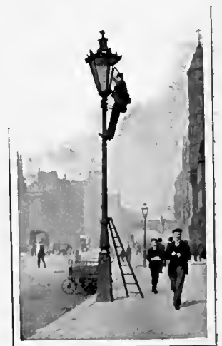
SUPPLYING ARC LAMP WITH CARBON.
