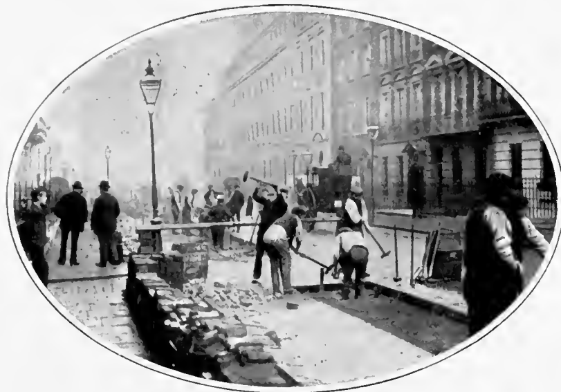
LAYING ELECTRIC CABLES.
