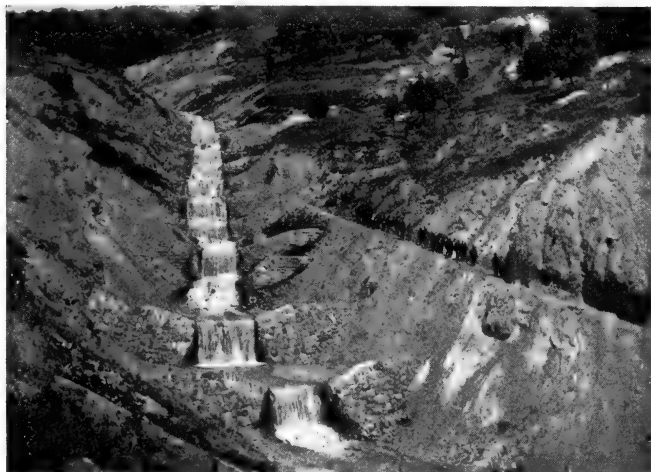
FIG. 46.—Masonry dams built to control a torrent. Students of the French forest school at the right. Alps of southern France.
