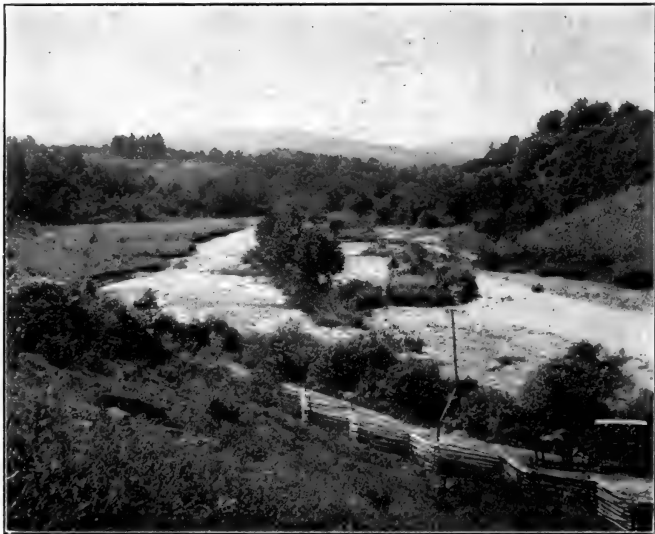
FIG. 45.—Destruction by flood. North Carolina.
