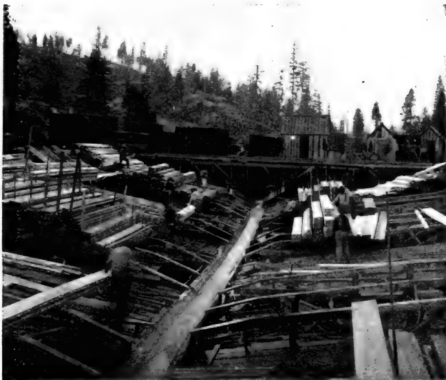
FIG. 1.—THE HEAD OF A LUMBER FLUME. CALIFORNIA.
