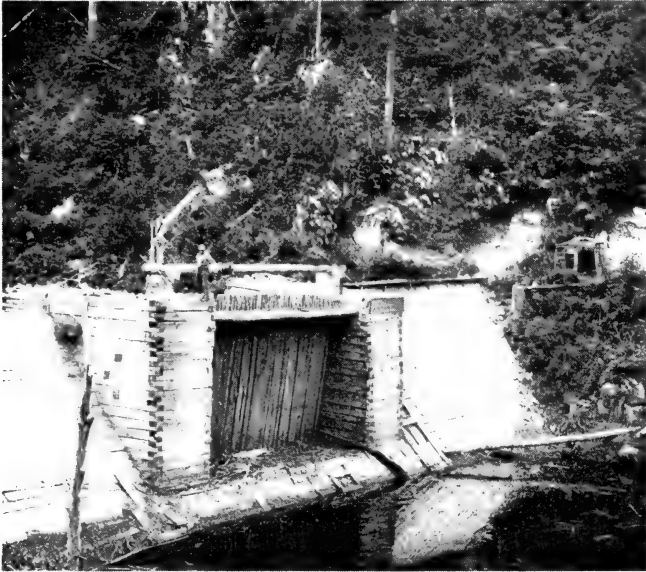
FIG. 1.—INTERIOR OF A SPLASH DAM. NORTH CAROLINA.
