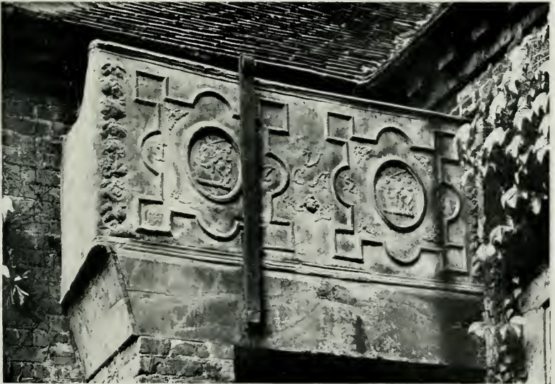
VERNON HOUSE, FARNHAM. LEAD CISTERN IN STABLE YARD.
